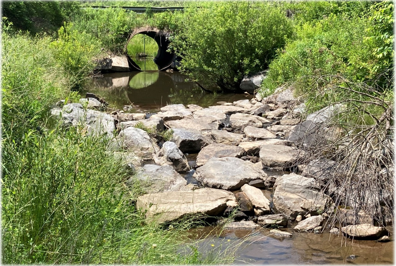
Figure 1. Engineered rock riffle below Pleasant Valley Rd on Spring Mills Creek, June 29, 2023.
