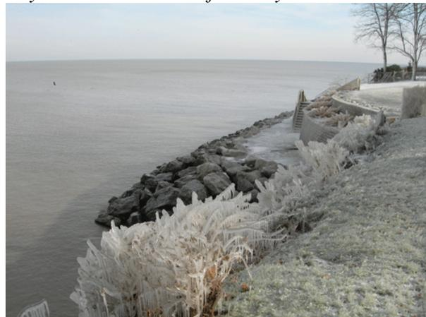
1. The material should be resistant to erosion caused by run-up and water washing through the armor stone. Fine grained material or a mix of larger material with fines should not be specified. *A revetment is shown in the above photo.*
