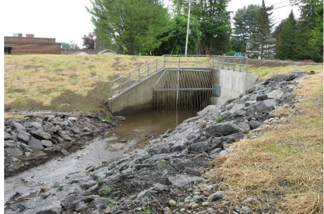
Above are an improved culvert and sidewalk crossing at a flood-control levee originally constructed in 1974. Many existing flood-control structures in the Mohawk River basin need upgrading and modernization to continue to effectively protect communities. Approximately $1.1 million in NY Works funding has or will be invested in these types of projects in the watershed.
