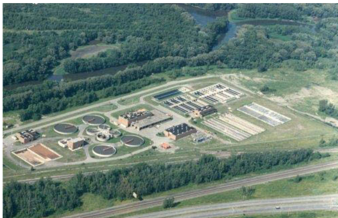
Above is the Oneida County Water Pollution Control Plant, located in Utica. The plant has an operating capacity of 48 million gallons per day and discharges to the Mohawk River. Oneida County and the NYS EFC have begun to invest significant resources in system upgrades which will improve Mohawk River water quality in the region. Photo courtesy of http://www.ocgov.net
