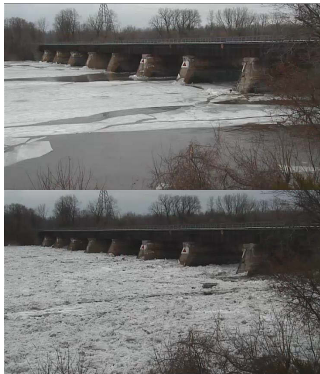
Images captured just 20 minutes apart by the project webcam show how quickly river conditions can change in response to ice jams. The camera is web accessible to the public and emergency managers during winter months to assess river conditions and related threats to public safety.
