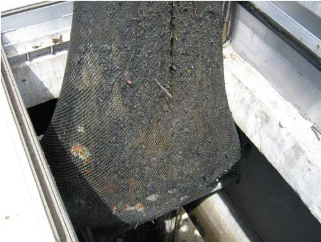
Figure 5. Net with Captured Floatables from Bronx River Floatables Control Facility
