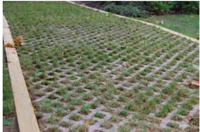
Figure D-I-2. Permeable pavement is a type of runoff reduction (RR) practice because it allows processes such as filtration and evapo-transpiration to occur. This approach reduces runoff and removes a greater portion of pollutants than stormwater treatment (ST) practices that employ a permanent pool – such as wet ponds, wet swales, and constructed wetlands – because such practices simply provide storage and treatment before discharge. Photo: Chesapeake Bay Program
