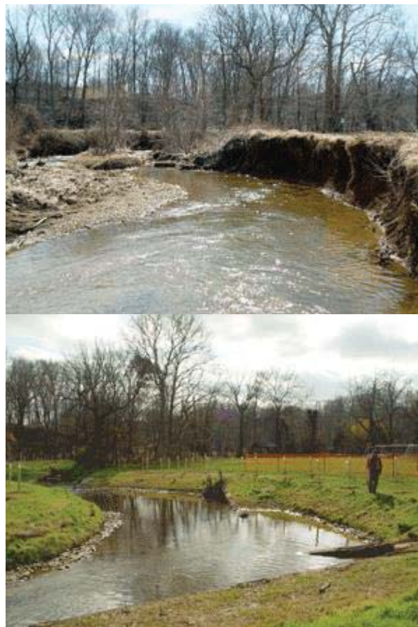
Figure A-9-1. Stream restoration projects can improve the health of aquatic resources and can be one of the more cost-effective practices to reduce nutrient and sediment loads in urban watersheds. A stream prior to restoration (top) that has an eroded stream bank and channel can be restored so that natural processes reduce the erosive energy of the stream flow during storm events. The bottom picture is the same stream shortly after completion of the project. Photos: US Fish and Wildlife Service
