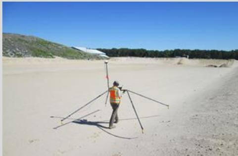
Electrical check for leaks in newly installed landfill liner in Cell 6 Phase XI prior to obtaining certification for construction, and commencing landfilling activities
