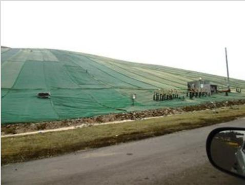
On long slopes, the Town installed temporary geosynthetic intermediate covers to prevent washouts during major rain events
