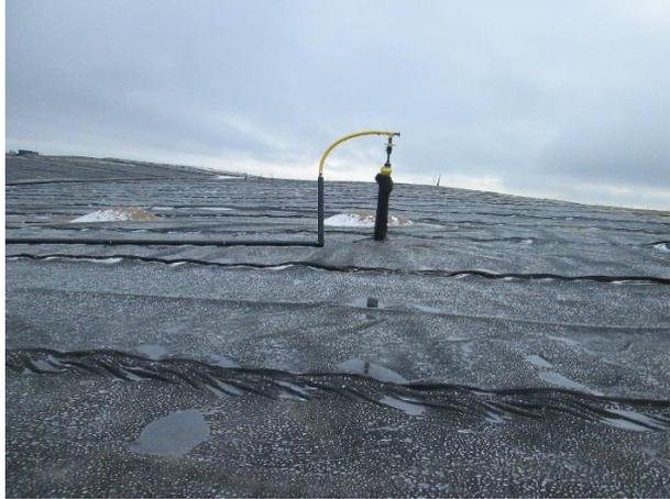
**Vertical Gas Extraction Well:** View of a completed gas extraction well after hook-up to the gas header pipes connected to the landfill gas flare system
