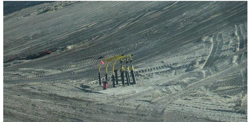
**Upgraded horizontal gas collection headers** connected to horizontal gas collection pipes at various elevations of the waste mass
