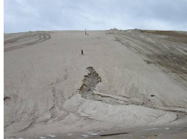
**Side Slopes:** View after washout of sand layer after a major rain event that plagued the cap project during the construction period
