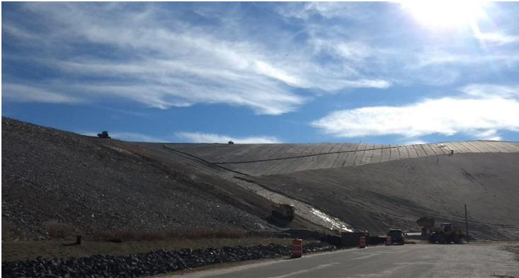
**View of the barrier protection layer:** using fresh sand to replace sand that was washed out by rain
