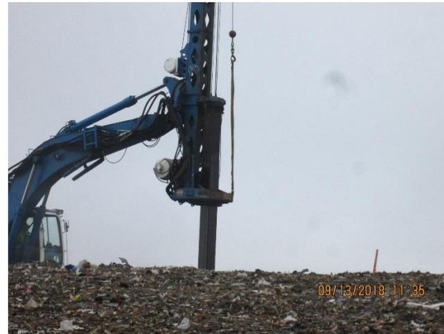
Drilling in the landfill mass to install landfill gas extraction wells, a critical component of the landfill cap design I component of the landfill cap design
