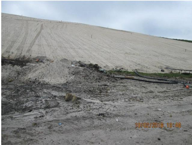
Side Slopes – View after placement of sand gas venting layer over graded waste
