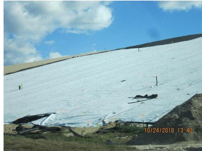
Side Slopes – View after placement of geo-composite layer
