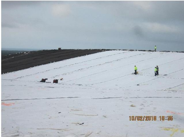
Top Area – View after placement of geo-composite layer
