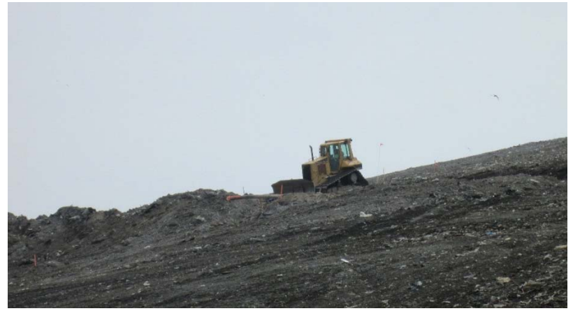
Close-up view of the side slopes being smooth graded
