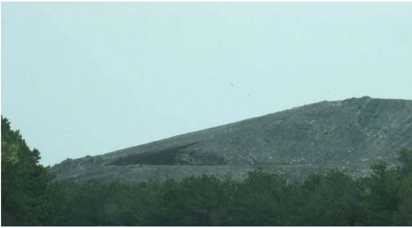
Smooth grading of side slopes as seen from Woodside Ave
