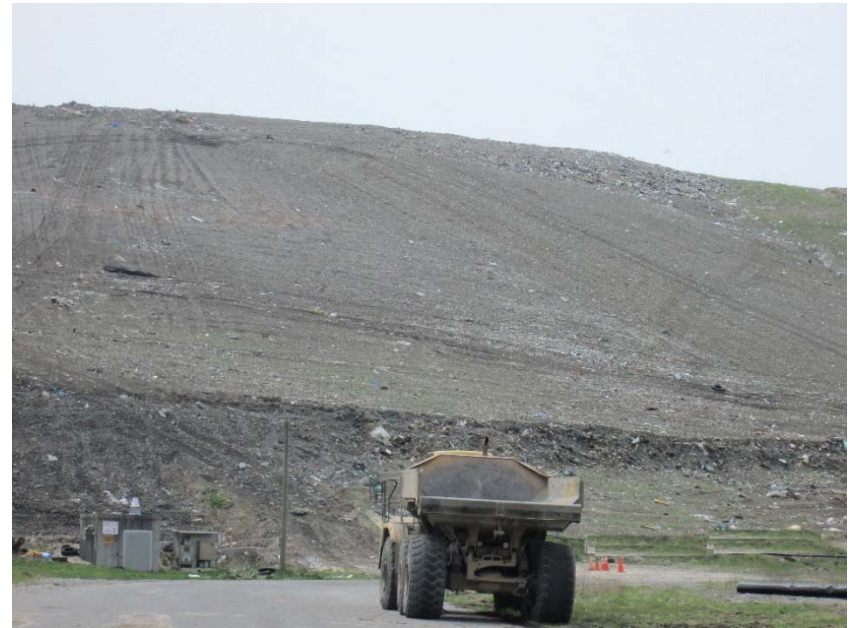
A section where smooth grading has been completed
