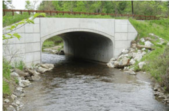
Good crossings that create no noticeable change in the stream include bridges and open-bottom arches and culverts that sufficiently span the stream channel bed, and box and pipe culverts that sufficiently span and are adequately sunk into the stream channel bed.
