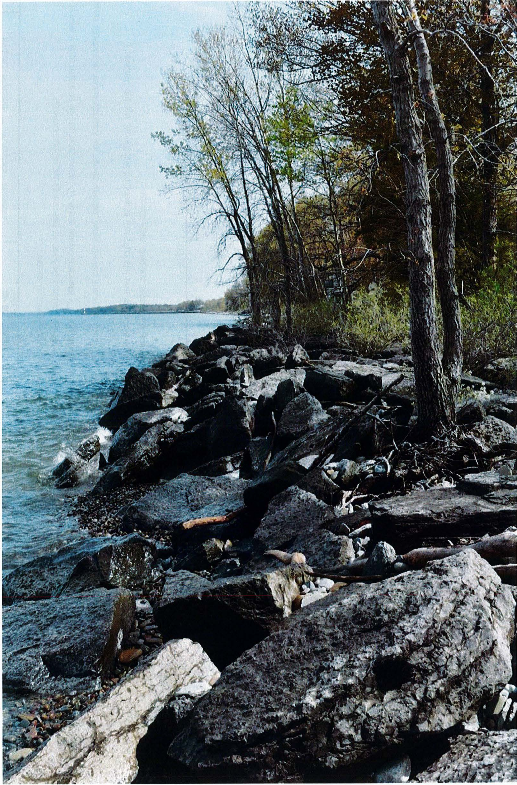
Photo 2. Shoreline protection along the banks of Selkirk Shores State Park in the 1960's and 1970's
