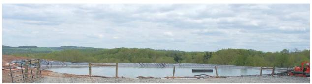
Photo 5.20 Fresh water supply pond. Black pipe in pond is a float to keep suction away from pond bottom liner. Ponds are completely enclosed by wire fence. Source: NYS DEC 2009.
