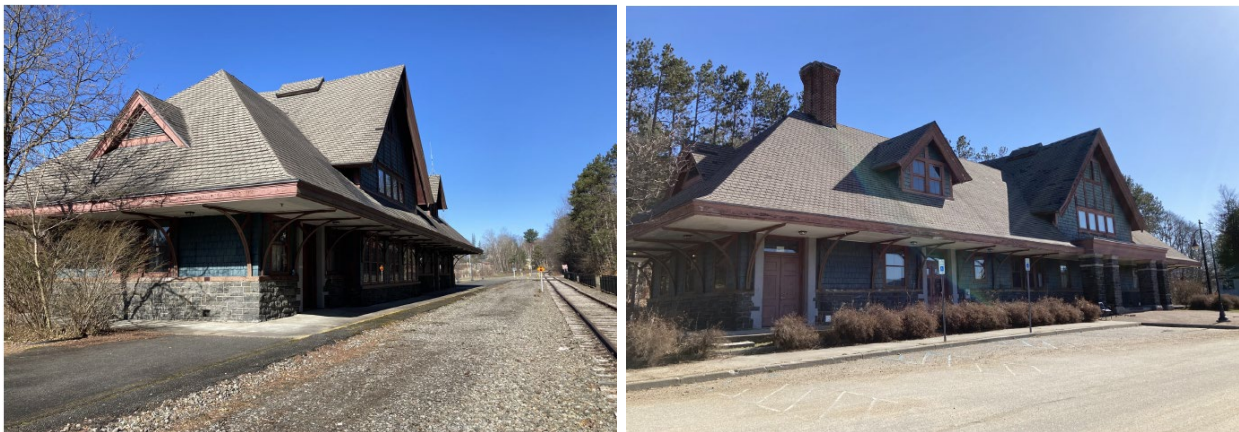
Figure 4: Current condition of Depot building (north and south sides).
