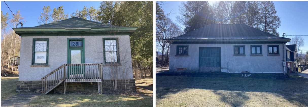
Figure 6: Current condition of Freight building (south and west sides).
