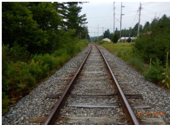
Typical Existing Ballast Track Section over Large Culvert
