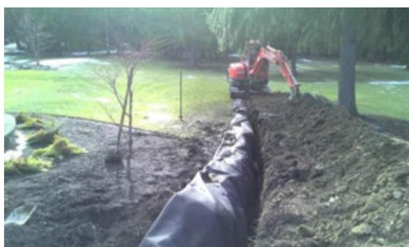
Root graft disruption barrier installed in Canandaigua to help prevent the spread of oak wilt.
