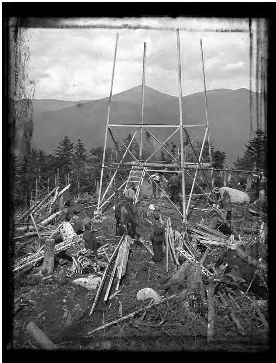
By 1916, New York State began building fire towers out of steel, which was more durable. Here a group of men, with the aid of horses, work to erect the tower on Mount Adams.
