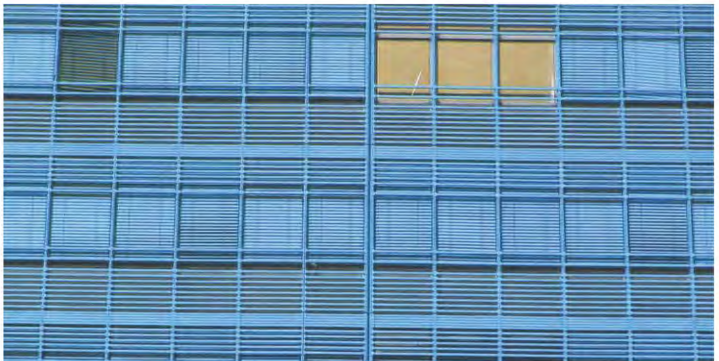
External screens or closely placed rods help keep birds from flying into glass.
