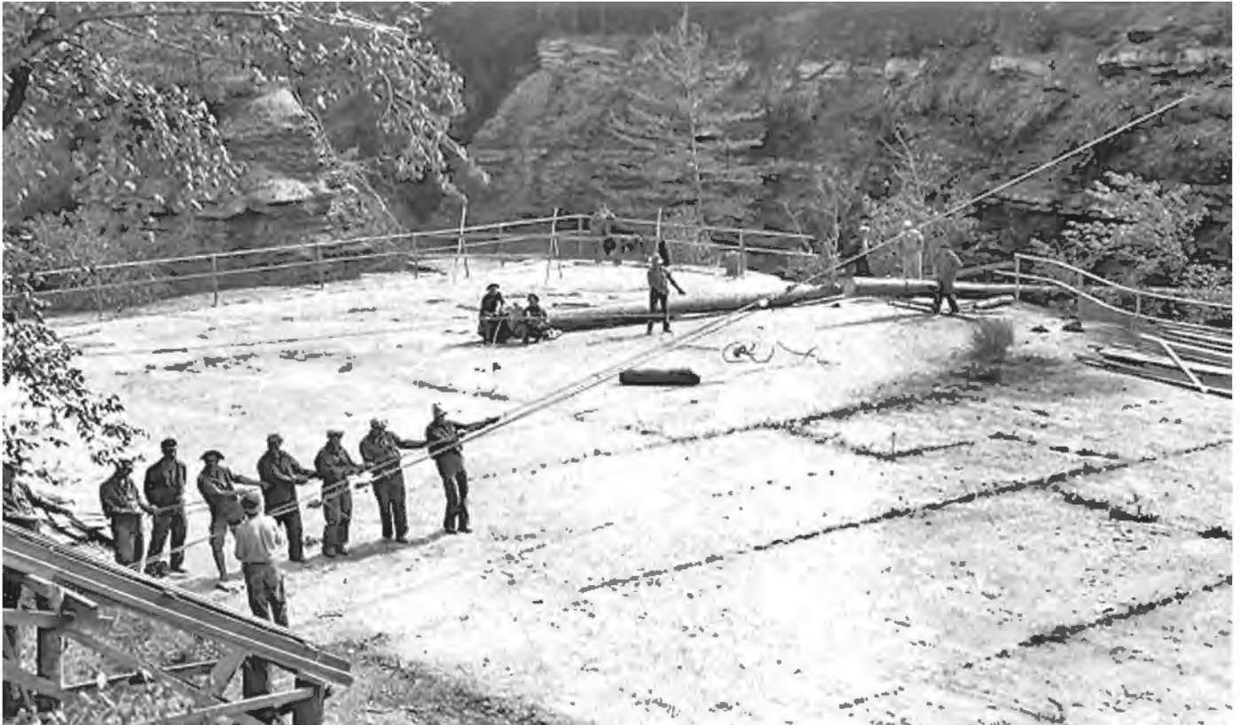
A CCC crew clearing trees on Table Rock at Letchworth State Park, in preparation for building what is now the Lower Falls Bridge.
