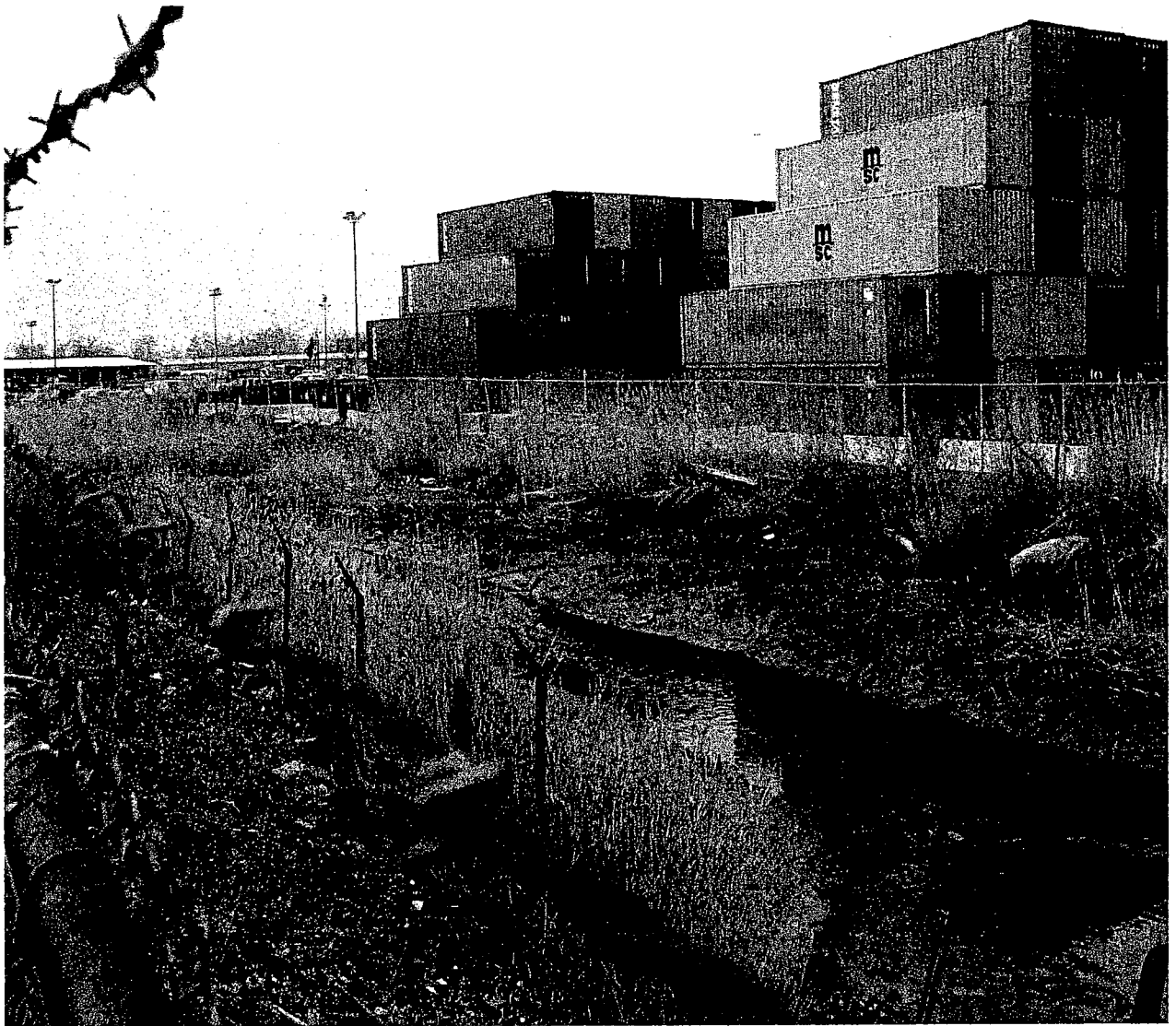
Port Ivory Intermodal Facility. Location of proposed bridge over Bridge Creek. View southwesterly. 4/04.
