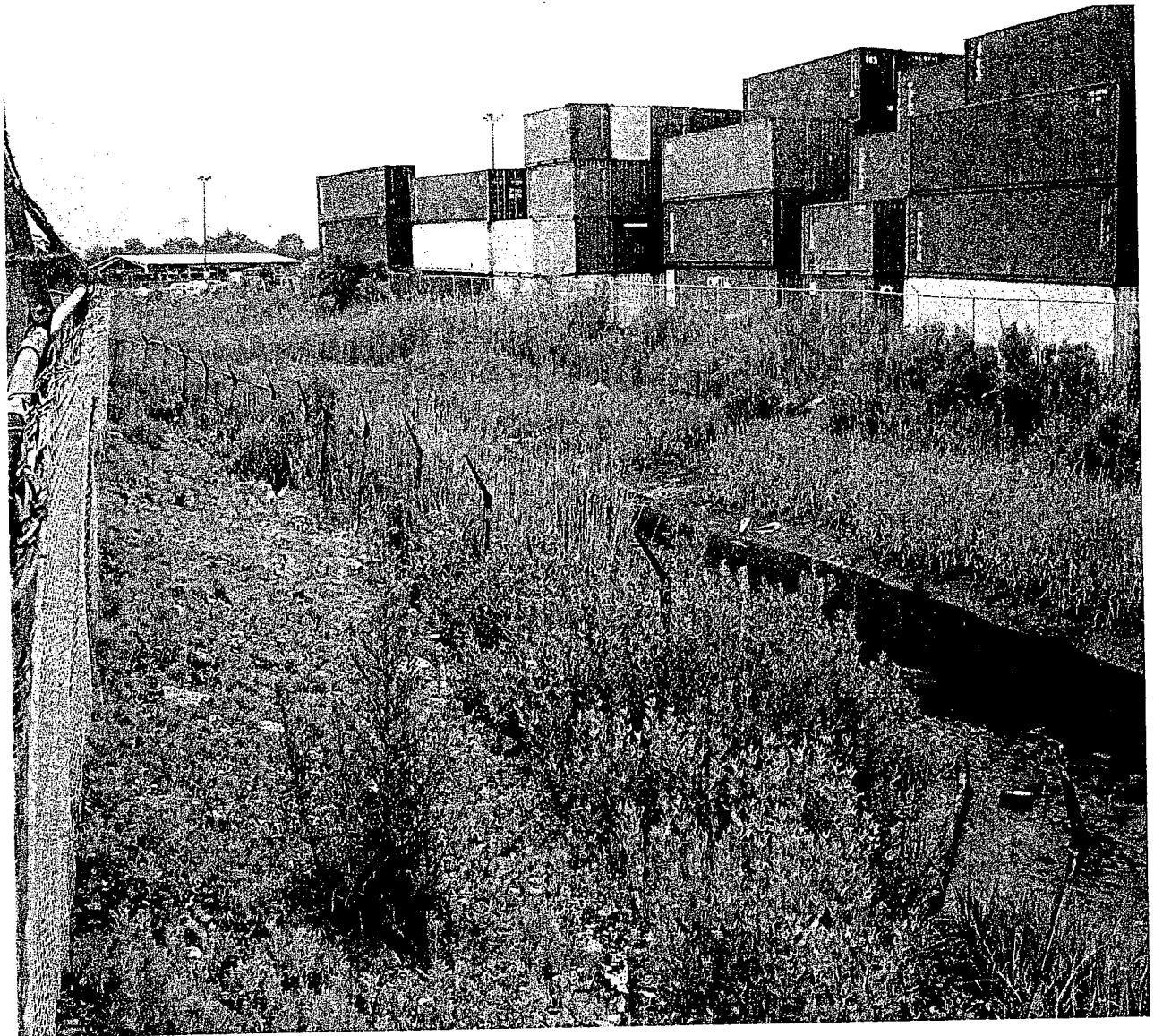
Port Ivory Intermodal Facility. Location of the bridge over Bridge Creek. View southwesterly. 5/04.
