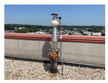
Photo 1: View of typical SSDS fan unit on the roof.
