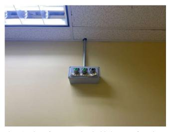
Photo 2: View of PMS associated with the SSDS fan units.
