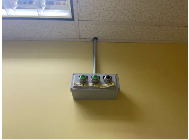
Photo 2: View of PMS indicating flow associated with the SSDS fan units.
