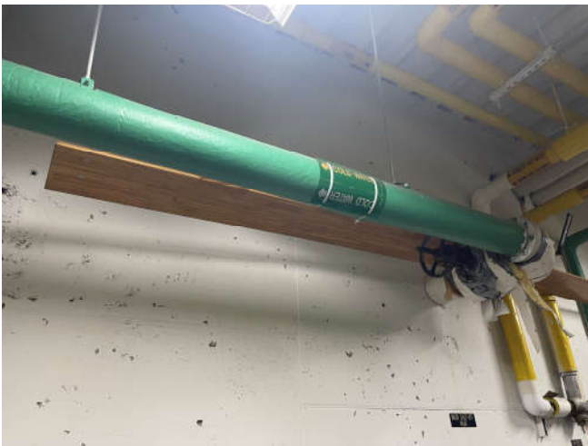
Photo 5: View of typical bare foundation wall in Room B24B.
