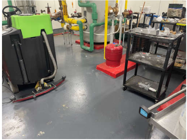
Photo 4: View of typical bare foundation floor in Room B24B.
