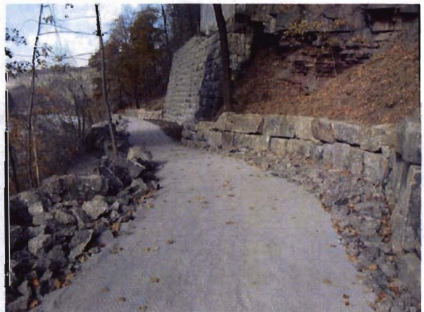
After – Looking North at Upper Retaining Wall
