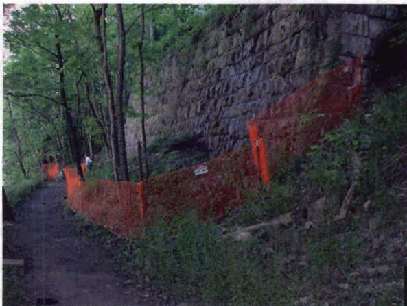
Before – Looking North at Upper Retaining Wall
