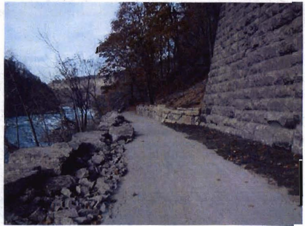
After – North end of Trail in Excavation Zone
