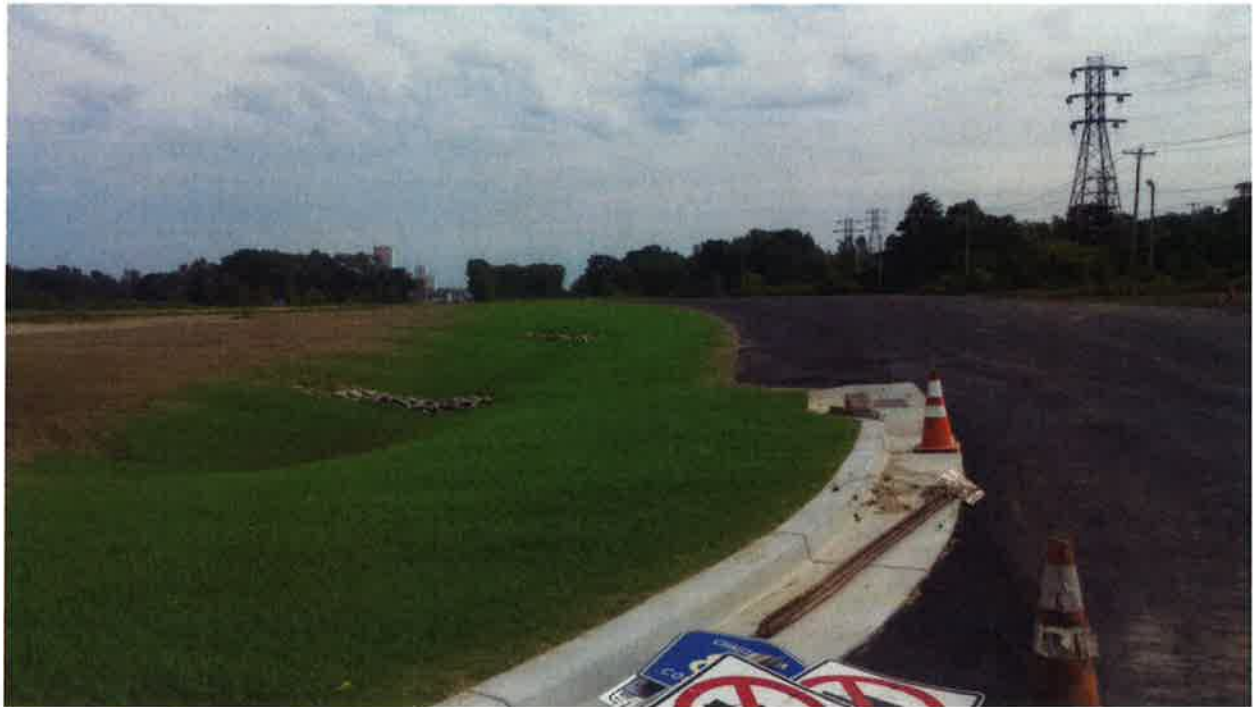
View of the completed roadway depicting that construction activities are complete
