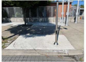
Photo 5: View of the repaired previously sinking light pole concrete pad.
