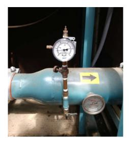
Photo 2: View of the newly installed blower outlet pressure gauge.
