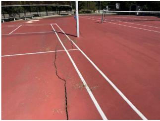
Photo 3: View of a typical previously existing crack on the tennis court.
