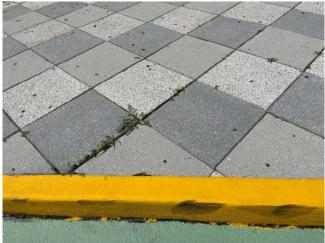
Photo 6: View of area identified as "loose pavers" with no cover compromised.
