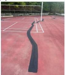
Photo 4: View of the recently sealed cracks on the tennis court.
