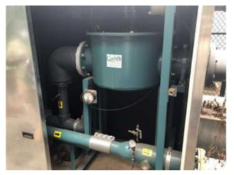
Photo 3: View of the SSDS fan unit.
