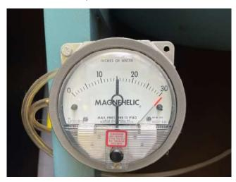
Photo 4: View of the SSDS vacuum gage.
