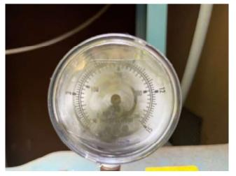
Photo 5: View of malfunctioned blower outlet pressure gauge.
