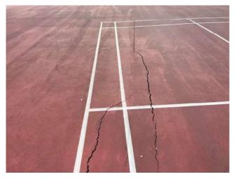
Photo 11: View of typical moderate crack on the tennis court.
