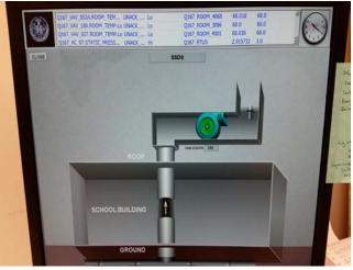
Photo 2: View of BMS connected to the SSDS fan unit (2017).
