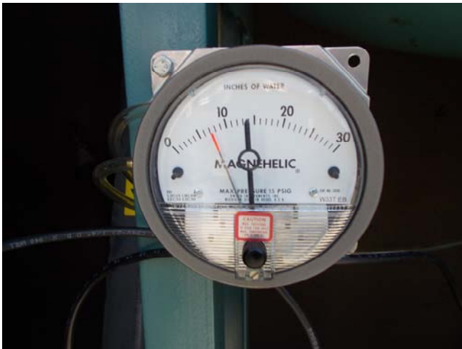
Photo 3: View of SSDS vacuum gauge.
