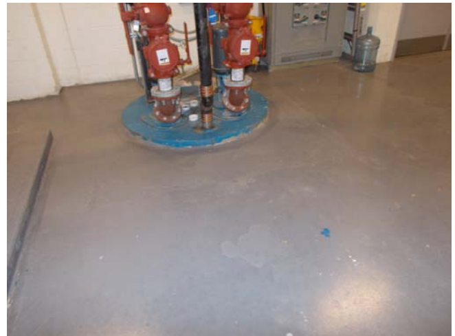
Photo 4: View of typical bare concrete floor (Room 0005).
