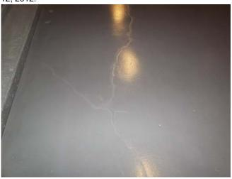
Photo 5: View of sealed crack in Room 0021.
