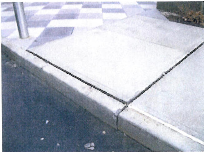
Photo 15: View of raised side walk and separation by Queens Metropolitan HS entrance.
