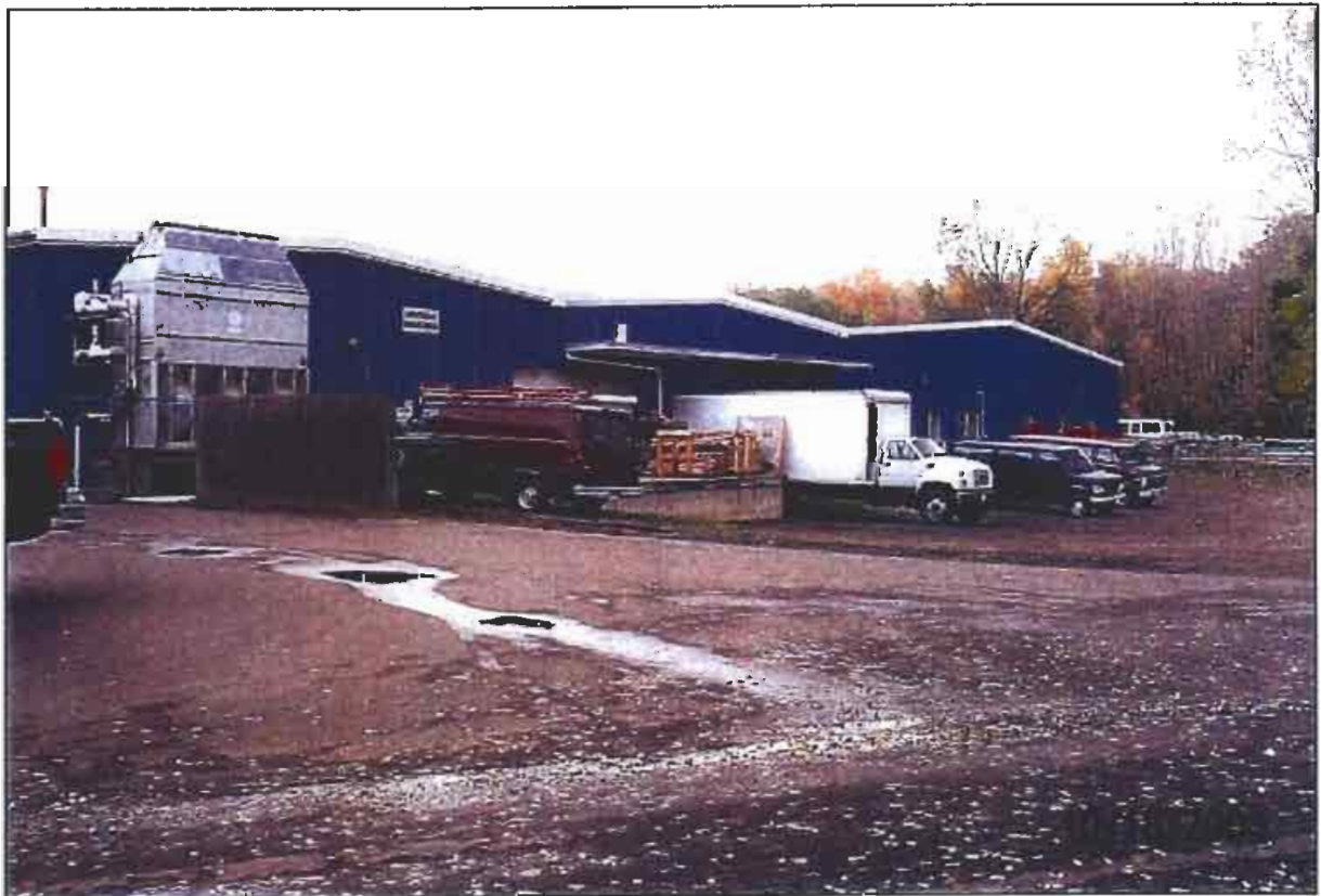
Photo 4 : West side of building, showing dock area.
