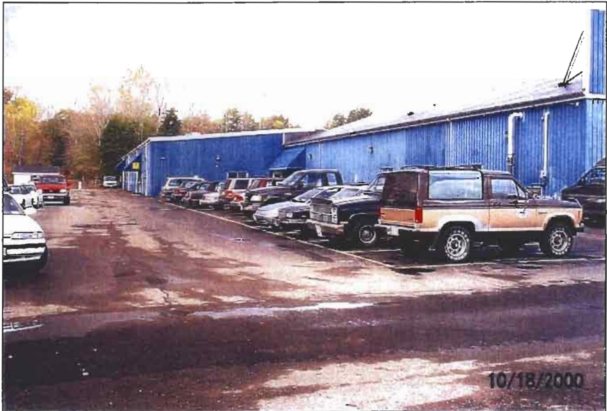
Photo 2 : View of south side of Day Center, looking west.
