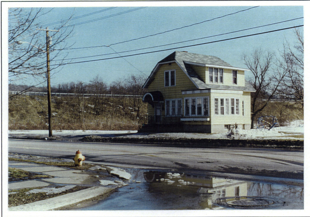
Photograph 1. View looking east of residence at 176 Central Avenue.
