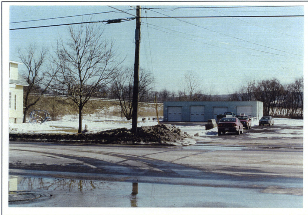
Photograph 2. View looking east of four stall garage behind residence.
