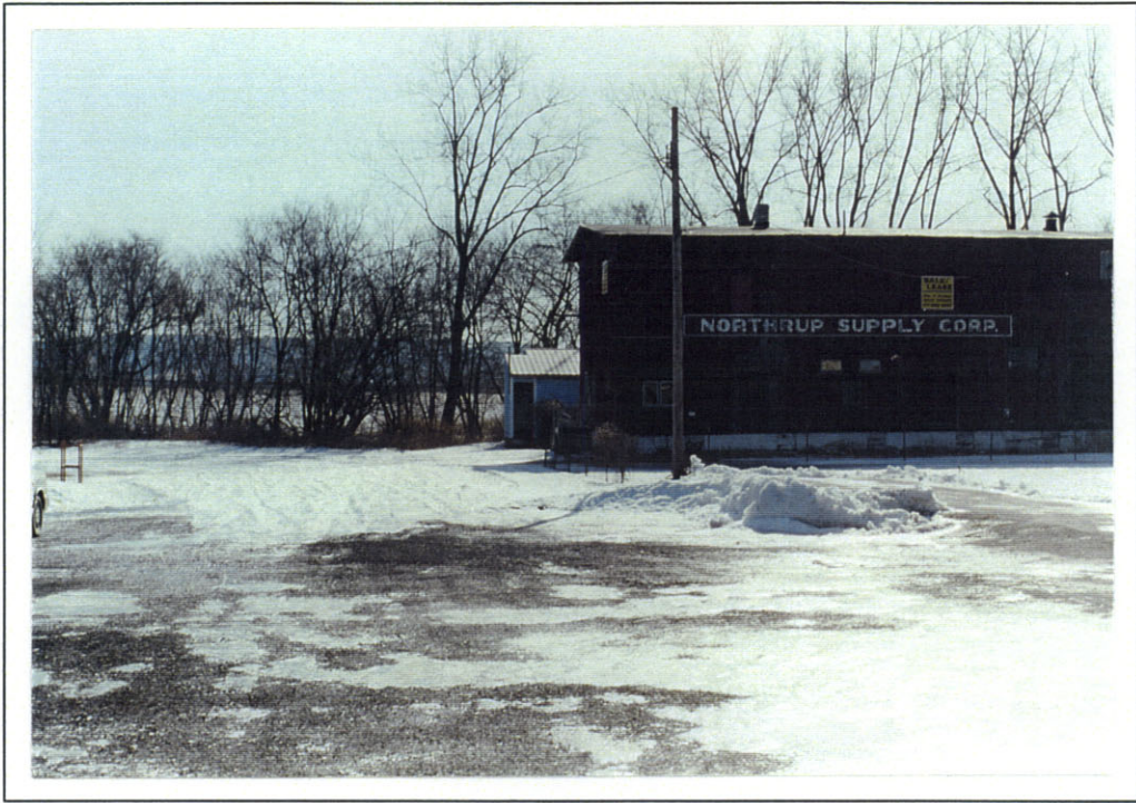
Photograph 3. View looking east of plumbing warehouse at 168 Central Ave.
