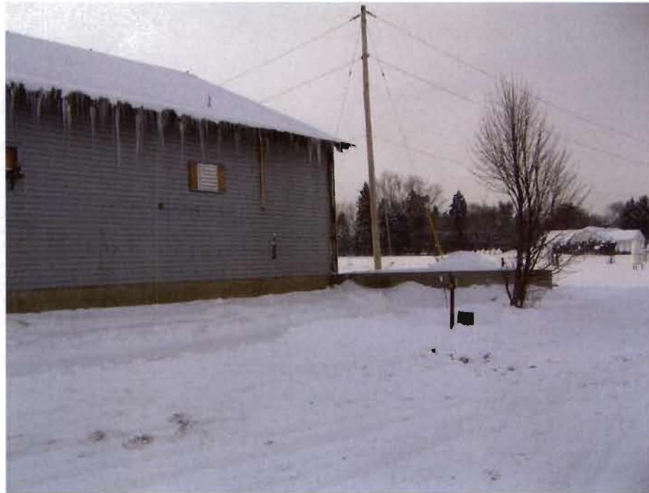
Photo 1: Site prior to start of excavation activities.
