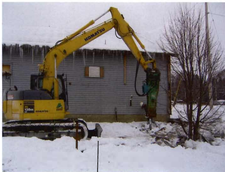
Photo 2: Demolition of concrete slab and former foundation wall.
