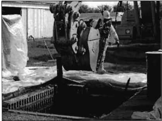
Sludge removal from the sump pit.
