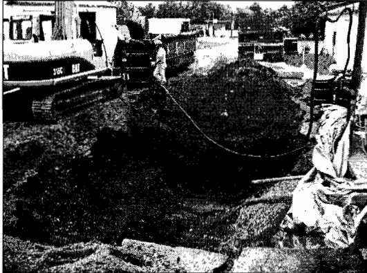
The final excavation, prior to backfill.
