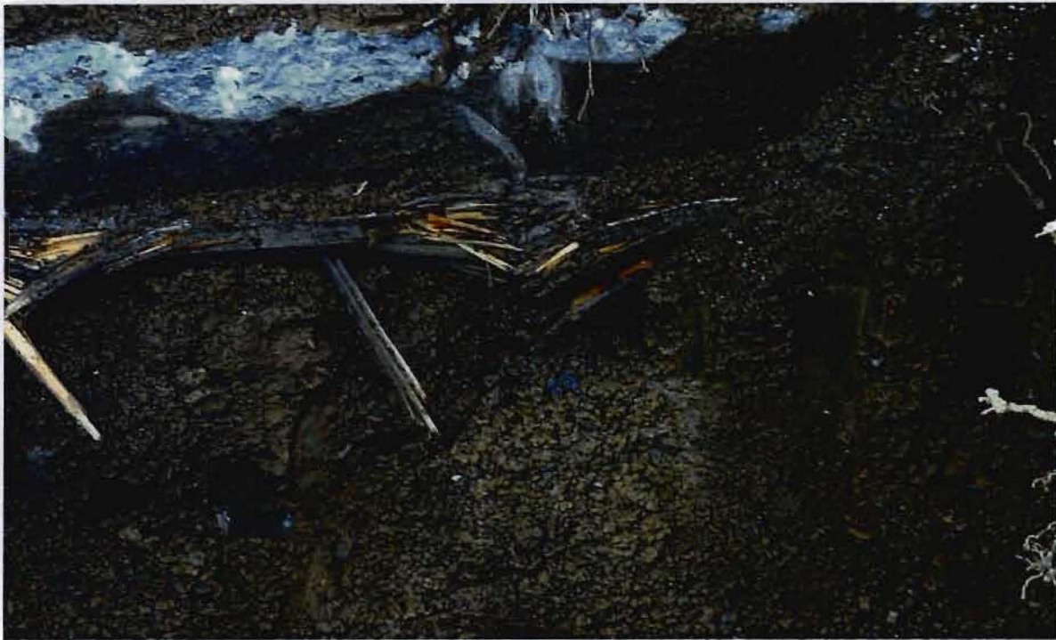
Southern wall after completion of 13 December 2000 remedial activities. Also the area of sample location PE-3.
