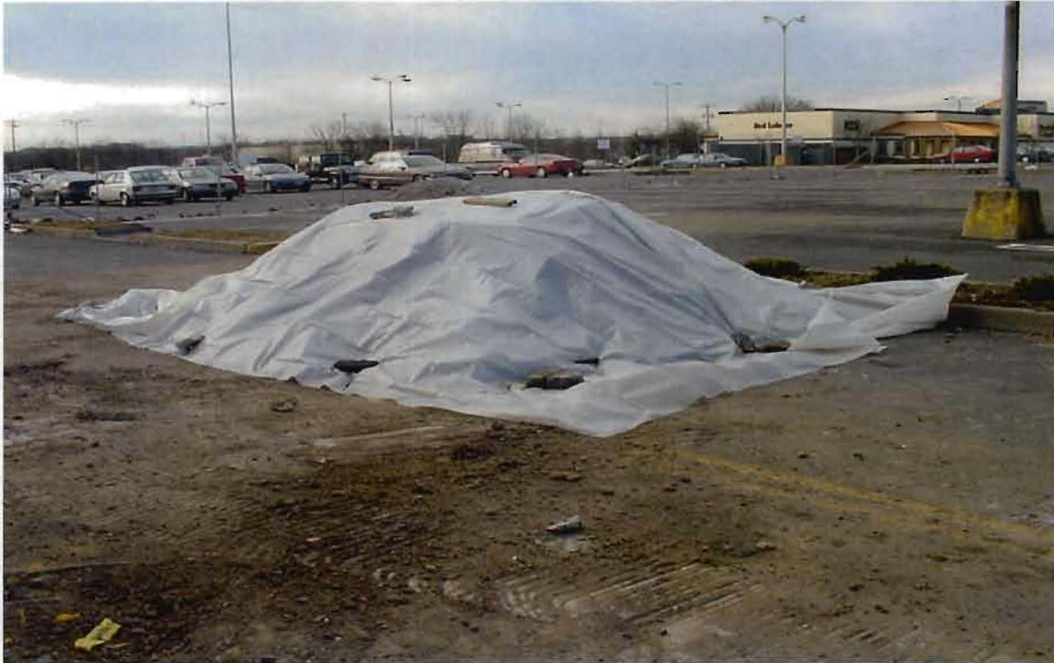
Remaining soils stockpiled after completion of 13 Decemeber remedial activities.
