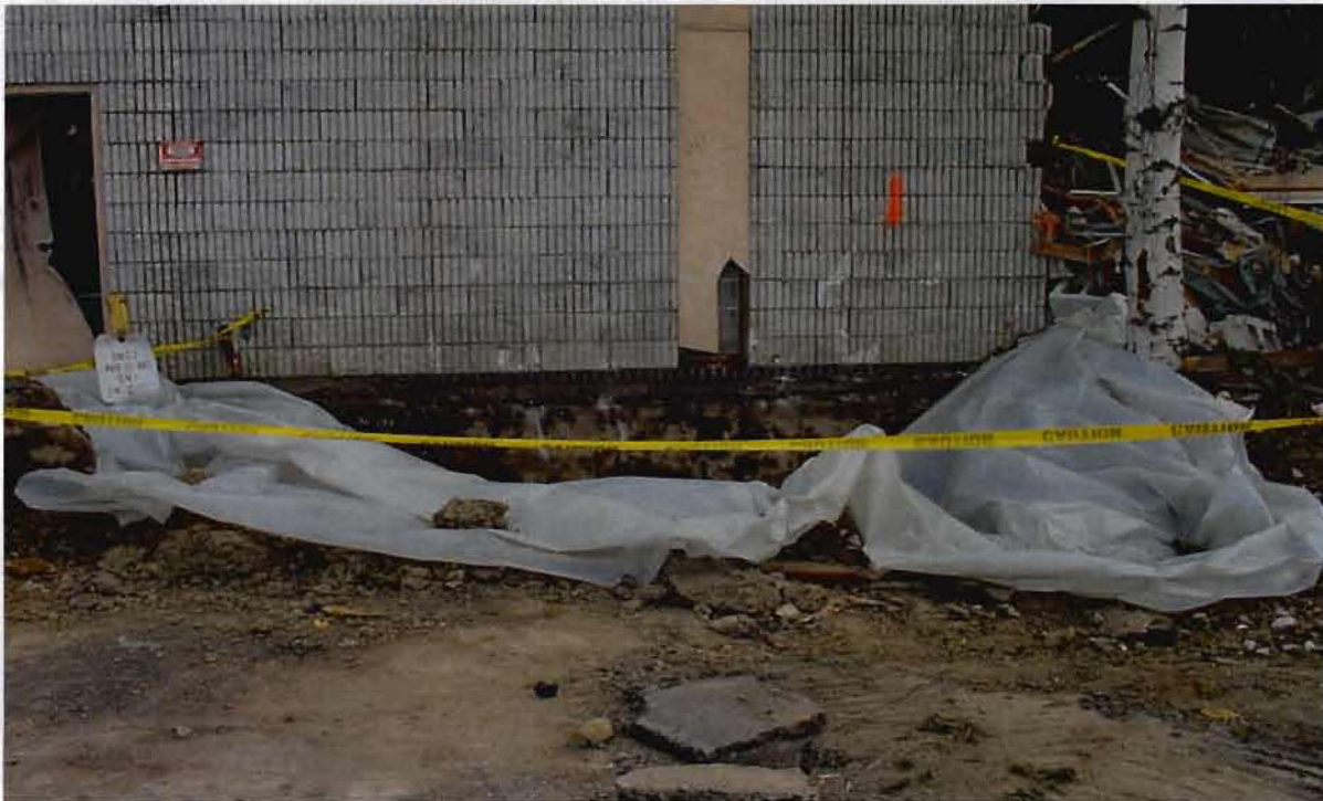
Excavation covered with plastic after completion of 13 December 2000 remedial activites.
