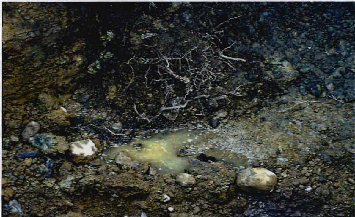
Western wall after completion of 13 December 2000 remedial activities. Also the area of sample location PE-1.
