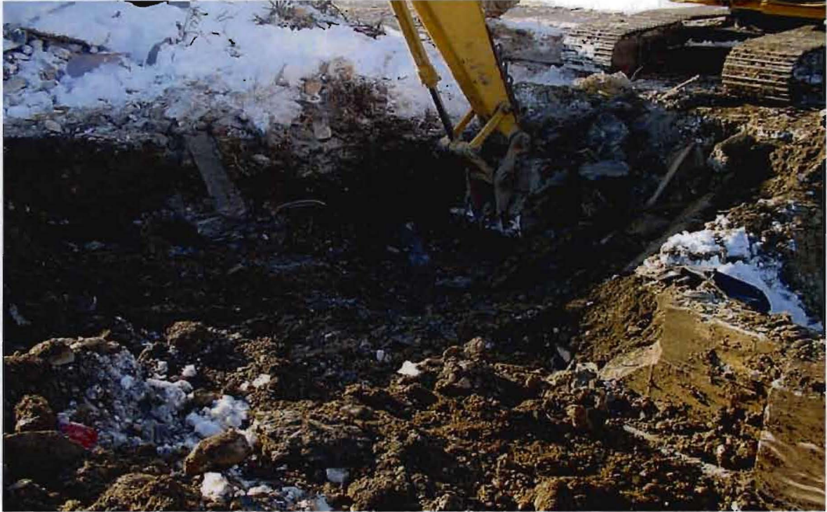
Concrete footing removed to access impacted soils.
