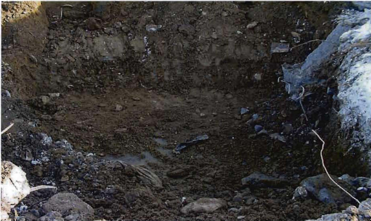
3 January 2001 excavated to a depth of seven feet below ground surface.
