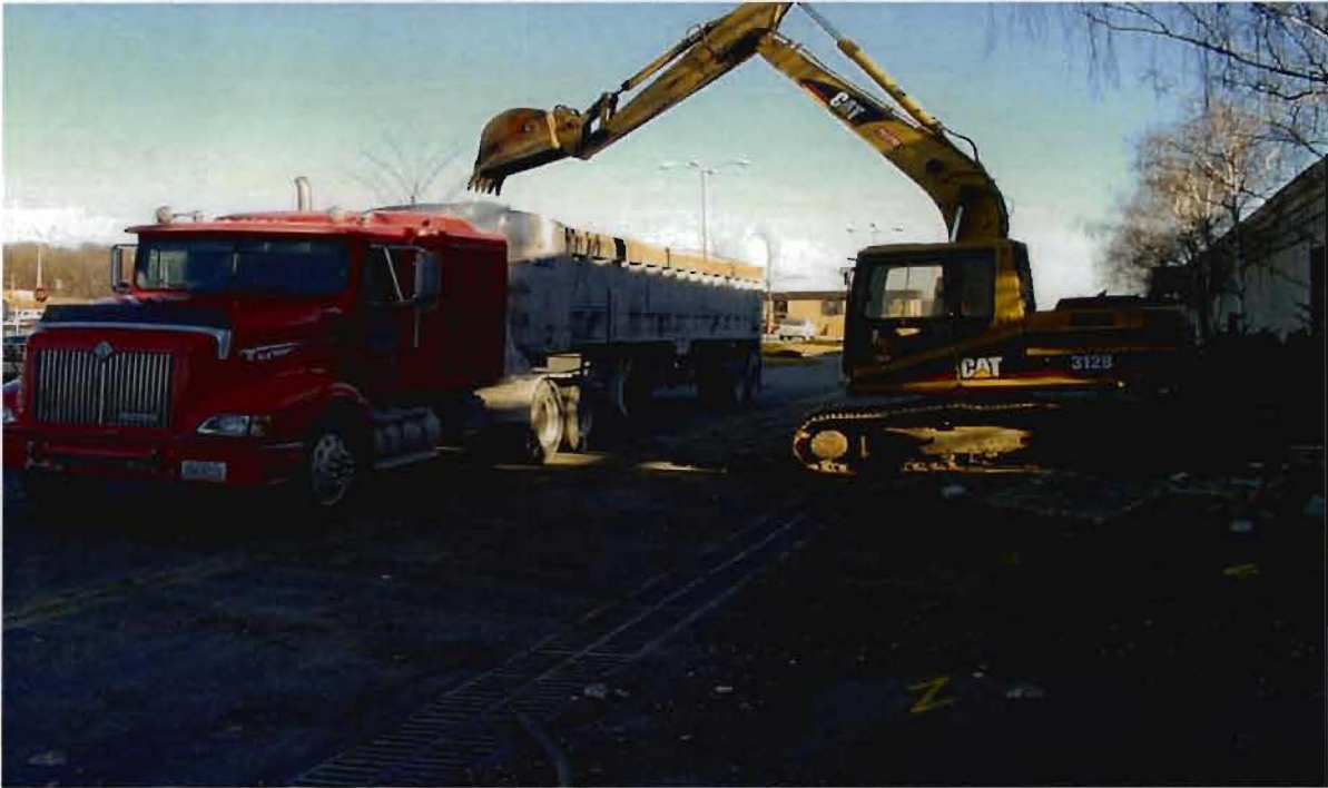
Loading of impacted soils during 13 Decmber remdial activities
