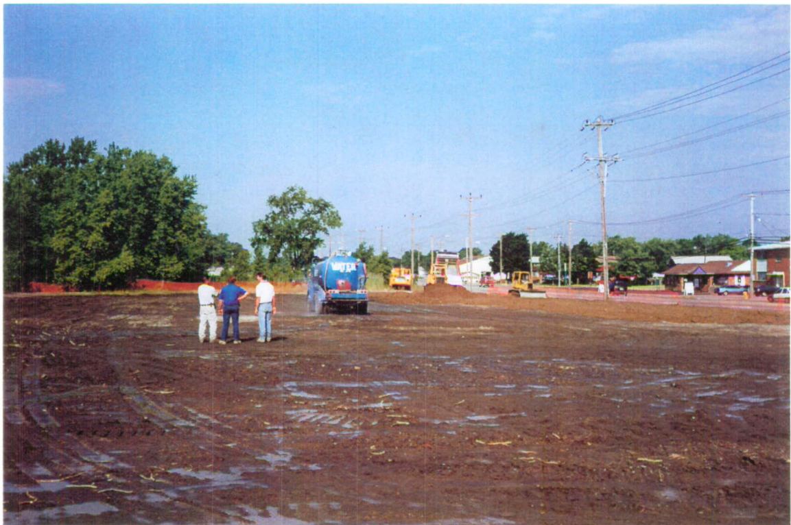
Topsoil receiving, July 15, 1999 Note how the lot is kept moist by the water truck
