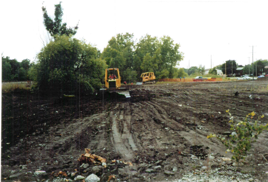
Initial grading of contaminated soil, July 13, 1999
