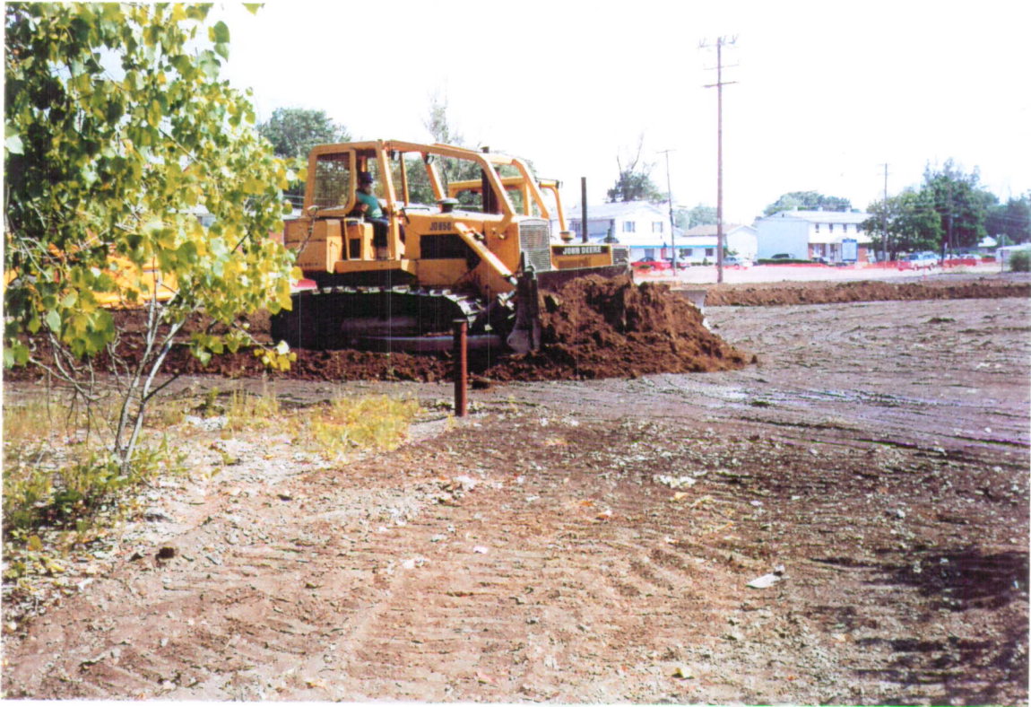
Grading topsoil over contaminated soil, July 15, 1999
