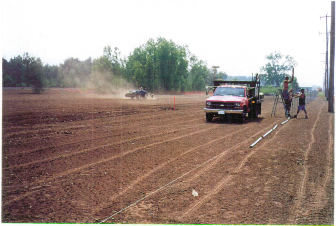
Rake out of topsoil and installation of fence, July 16, 1999
