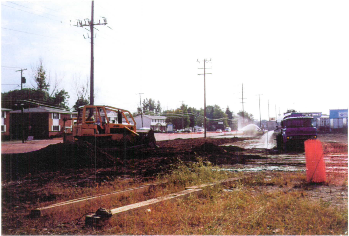
Topsoil receiving area at new entrance Water truck in operation, July 15, 1999
