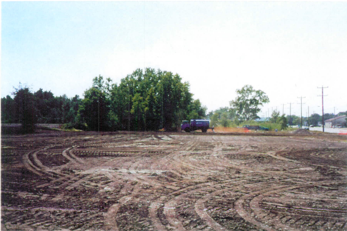
Rough graded topsoil end of July 15, 1999 Water truck still in operation
