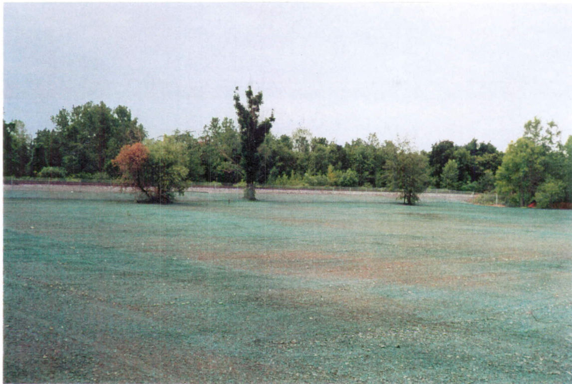
Topsoil surface hydroseeded, July 22, 1999
