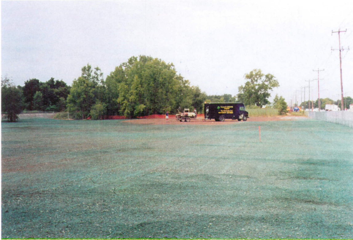
Hydroseeding equipment in operation, July 22, 1999
