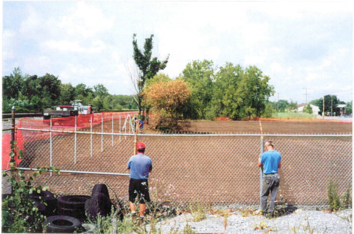
Repair to old end fence Installation of new fence, July 20, 1999
