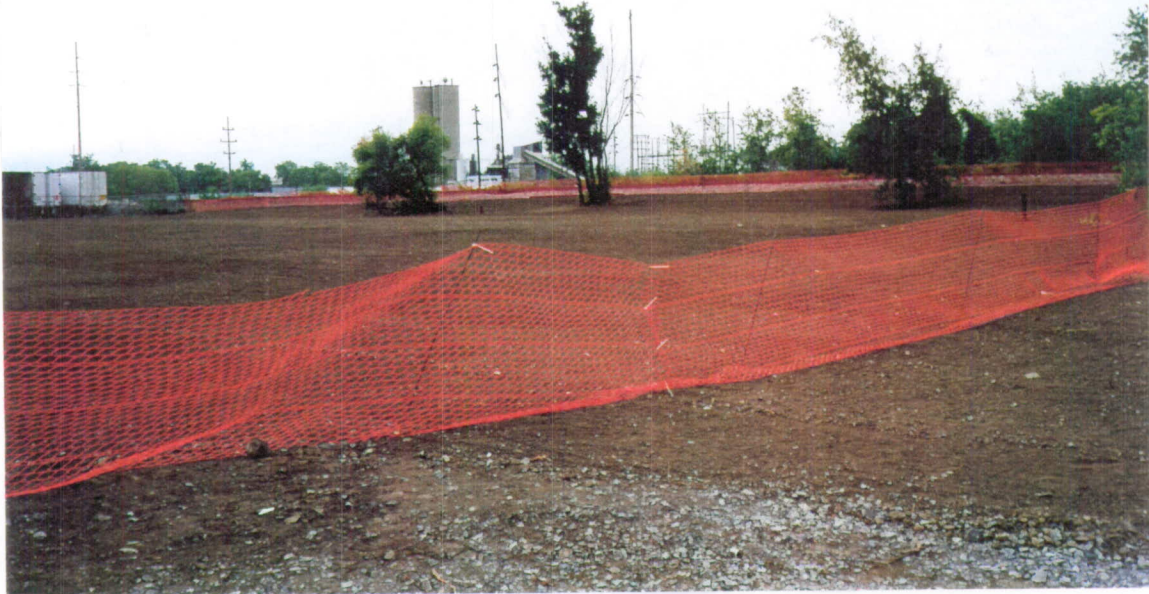
After rake out of new topsoil Safety fence in place, July 16, 1999
