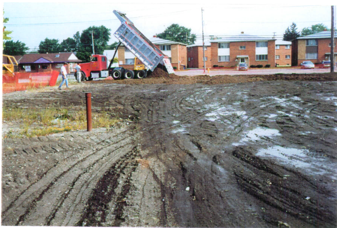
Receiving topsoil and water sprayed on the contaminated soil
