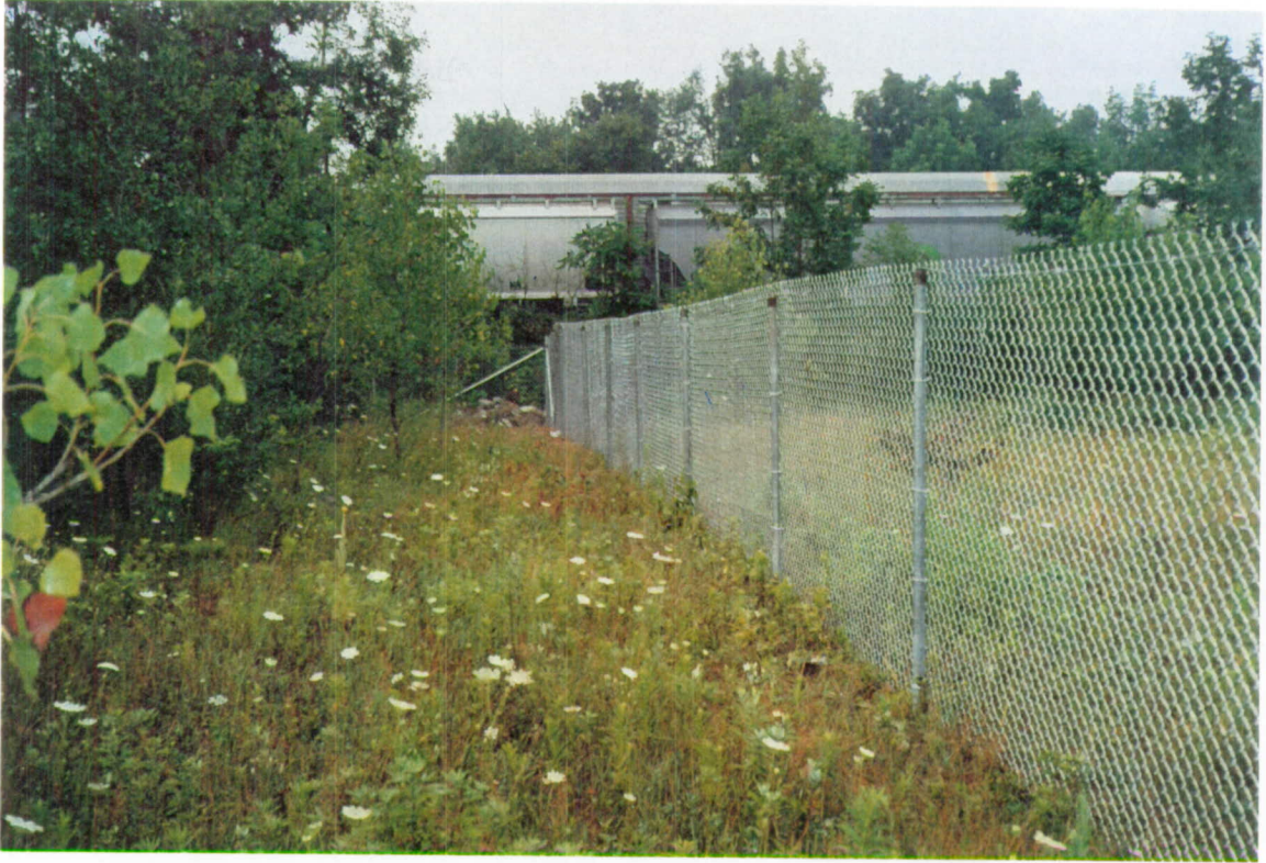
New fence across west end of work area, July 23, 1999
