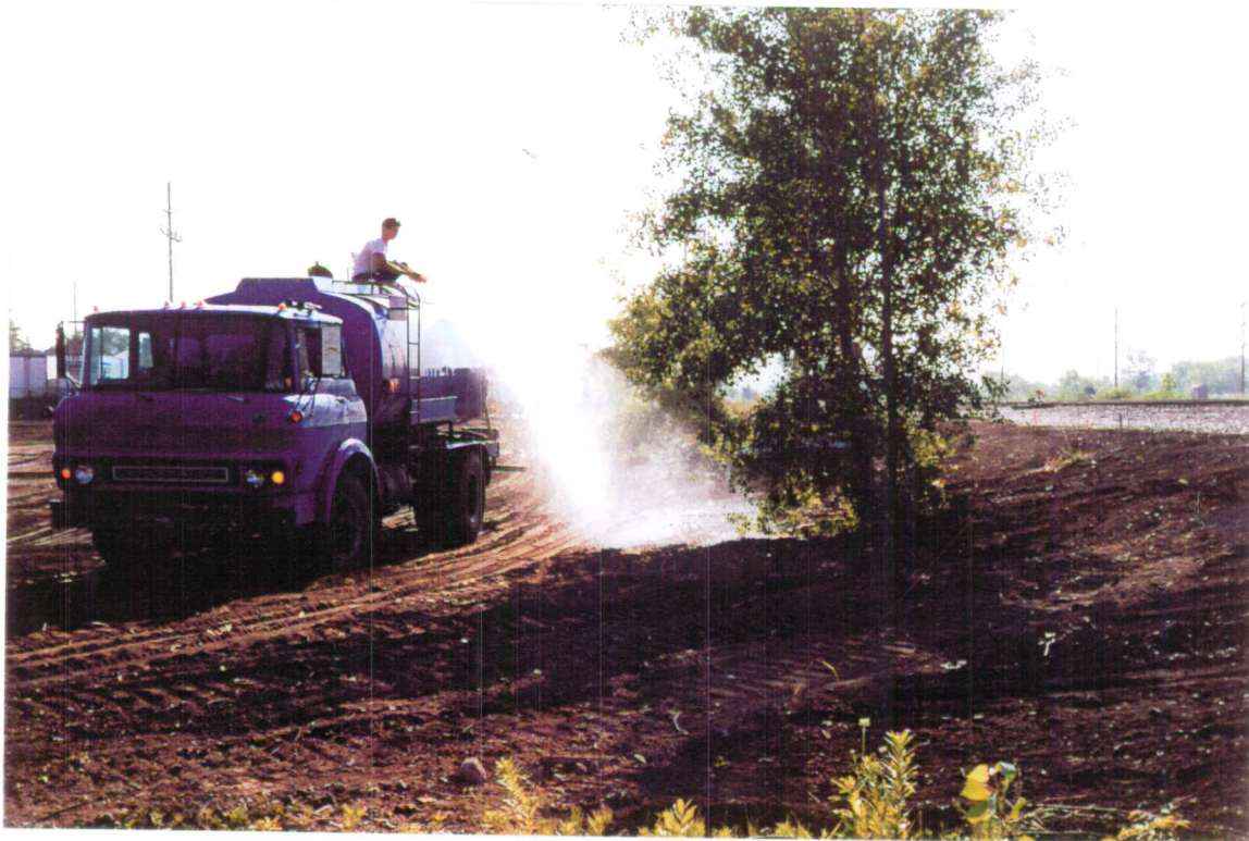
Water being applied to new topsoil, July 15, 1999
