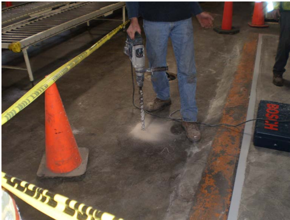
120909-02 SSV Monitoring boring.JPG
