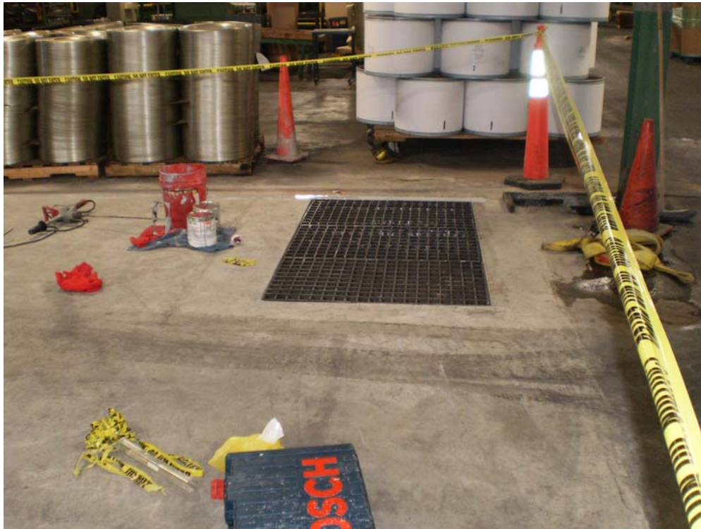
120909-01 New Vault grate.JPG
