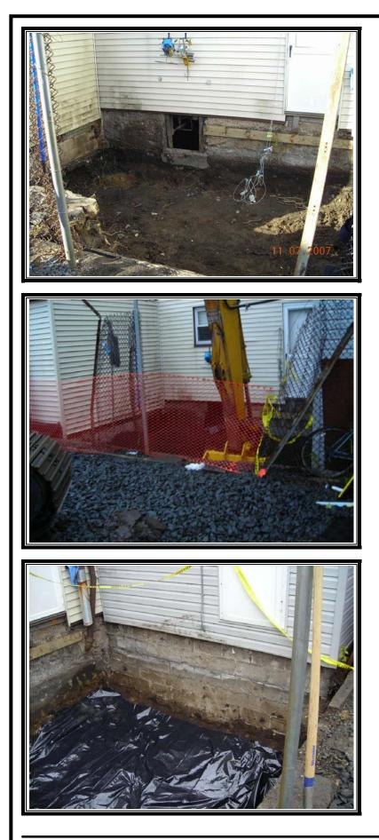
**Photo 1** – View of 57-42 after using Vactron to remove top one foot of soil in November 2008.
