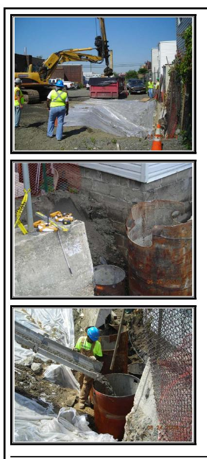
**Photo 7** – Disposal of soil from overdrill behind 57-42 into onsite container.
