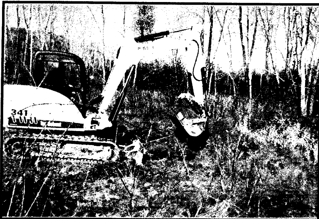
PHOTOGRAPH NO. 6 Test Pit 5 – Soil Excavation
