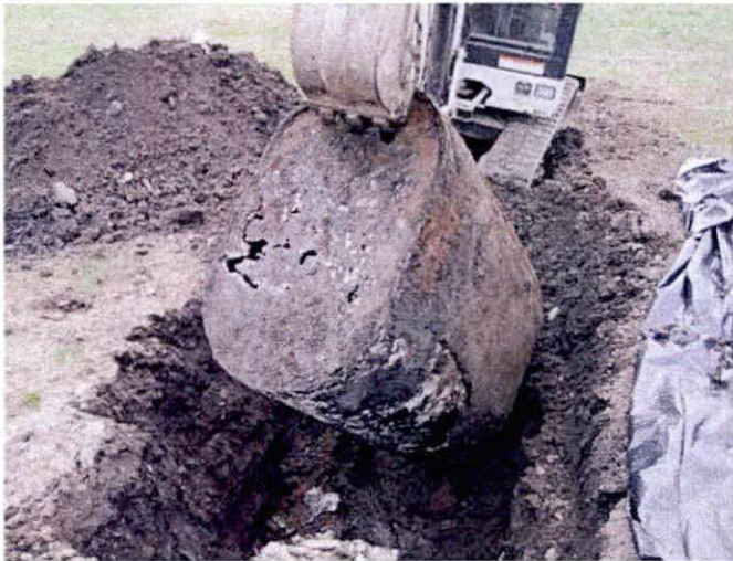
UST being removed. Note: Holes in side of tank – April 5, 2010
