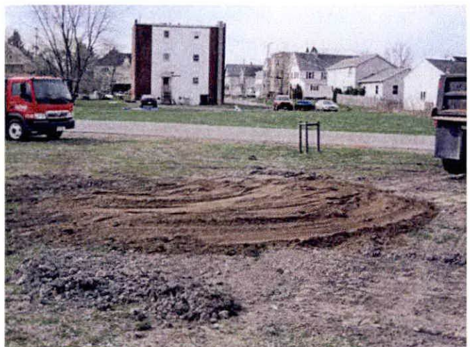
Completion of excavation
