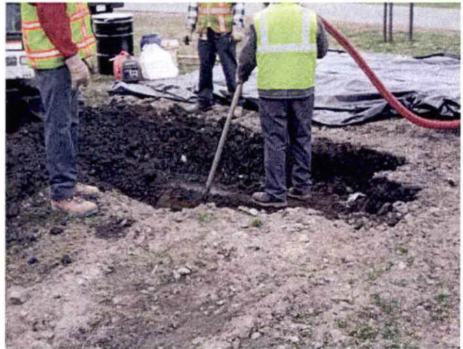
Removing the water/fuel oil mixture from the UST
