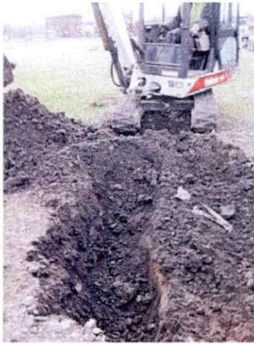
Uncovering the UST
