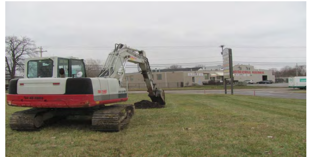
20. Test pit TP-7 facing east
