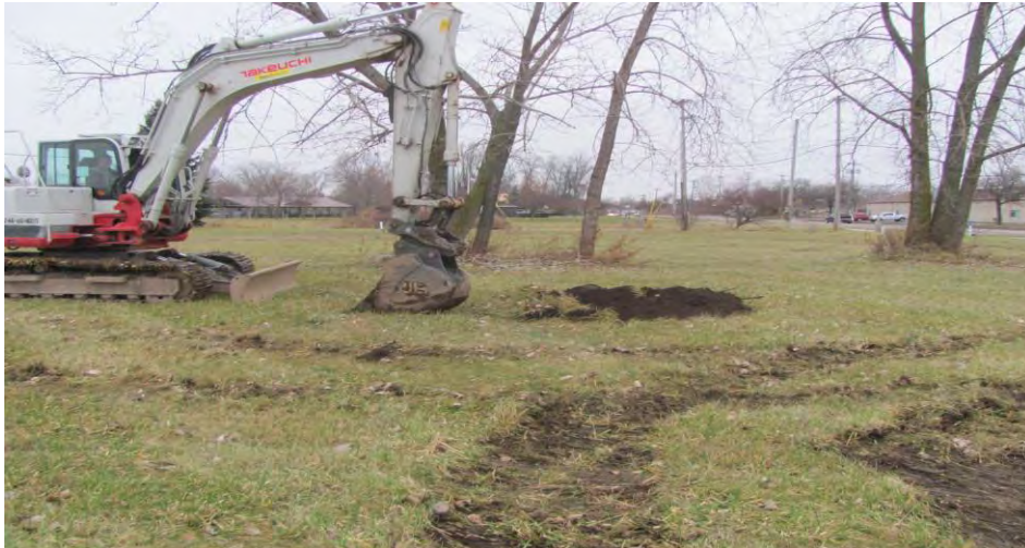
23. View of Test Pit TP-8 facing north
