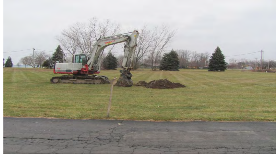
14. Location of TP-5 facing north
