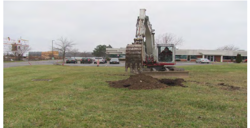
8. Location of Test Pit TP-3 facing west
