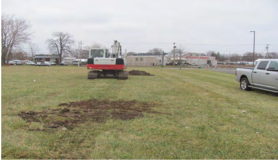
13. Location of test pit TP-5 facing east
