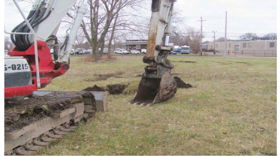
26. Location of Test Pit TP-9 facing east
