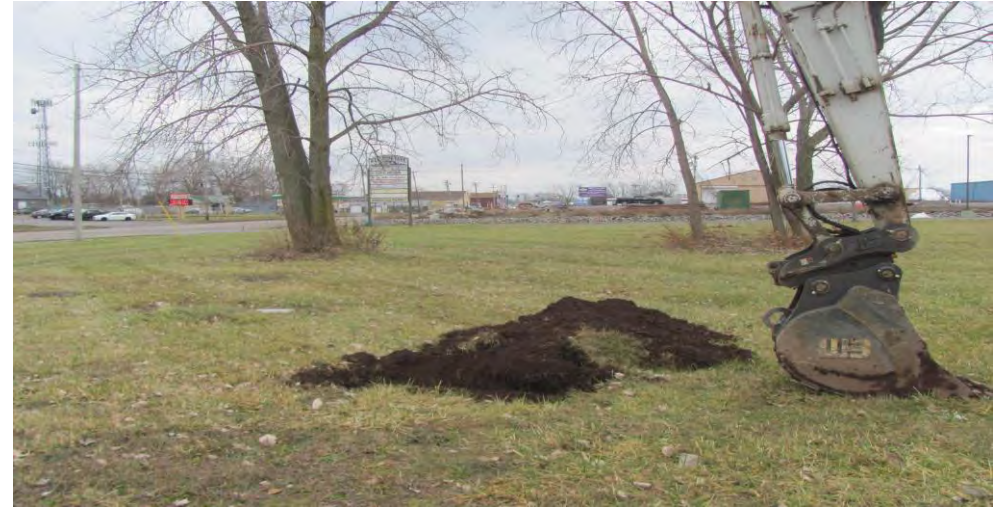
50. Location of Test Pit TP-17 facing south
