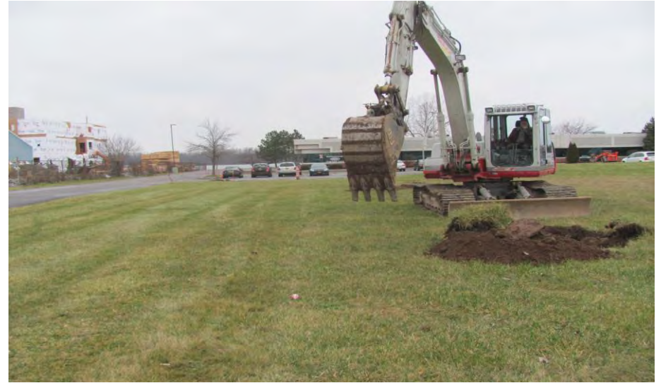
10. Location of test pit TP-4 facing west
