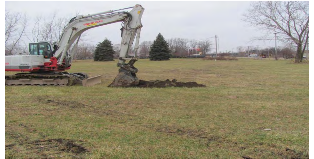
18. TP-6 facing north
