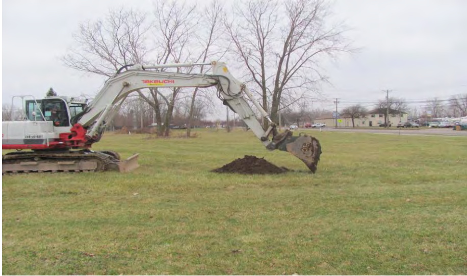
21. BH-7 facing north
