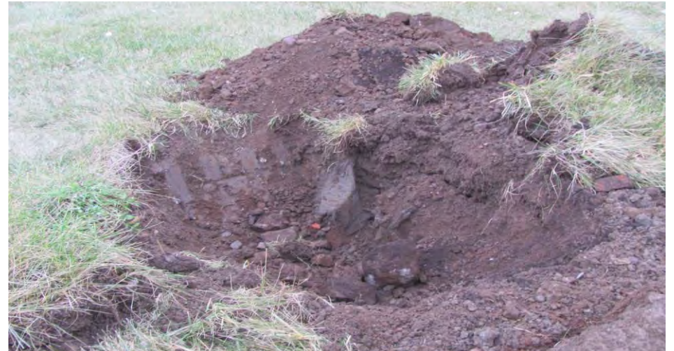
12. Test Pit TP-4
