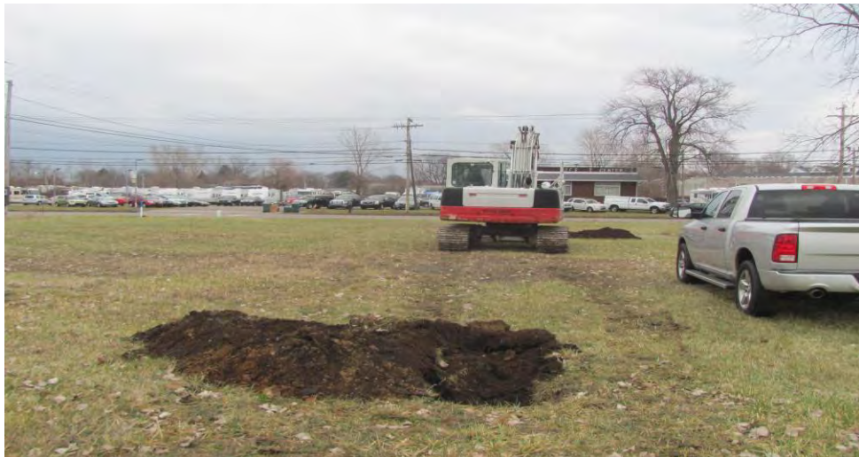
47. Location of Test Pit TP-16 facing east
