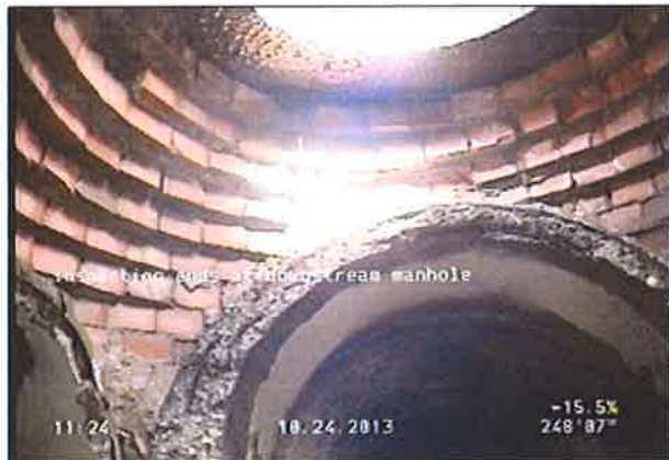
Photo: 10-9_10-10-6_22_24102013_112927_A.JPG inspection ends at downstream manhole
