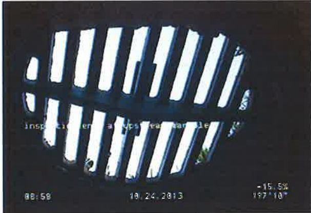
Photo: 10-8-21_10-9_12_24102013_090400_A.JPG inspection ends at upstream manhole
