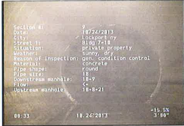
Photo: 10-8-21_10-9_1_24102013_083813_A.JPG inspection begins at downstream manhole / light steam and flow
