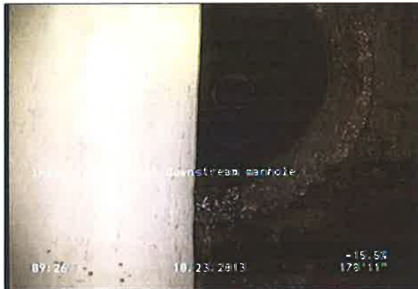
Photo: 10-3_10-4_19_23102013_093200_A.JPG inspection ends at downstream manhole
