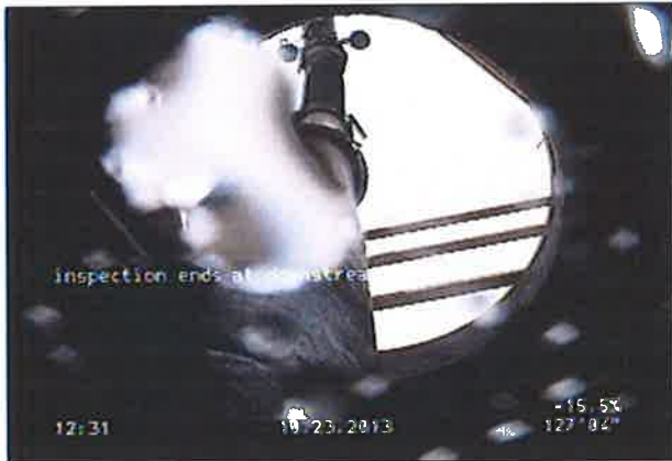
Photo: 10-5-7_10-7-21_12_23102013_123650_A.JPG inspection ends at downstream manhole
