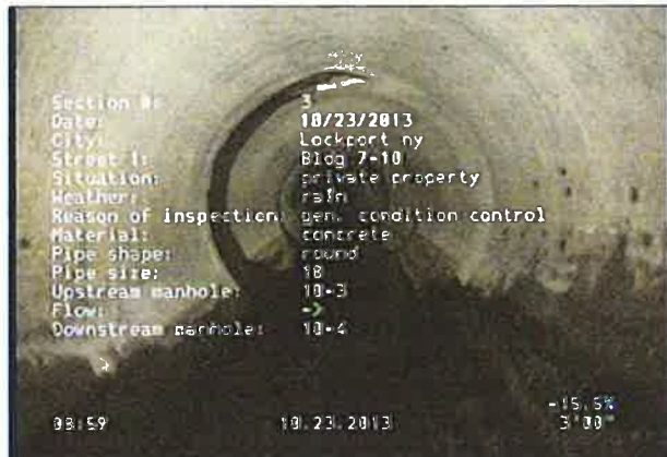
Photo: 10-3_10-4_1_23102013_090507_A.JPG inspection begins at upstream manhole / light flow
