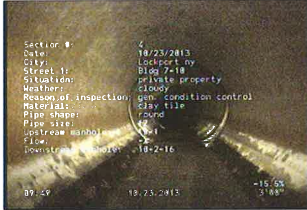
Photo: 10-1_10-2-16_1_23102013_095507_A.JPG inspection begins at upstream manhole / light flow
