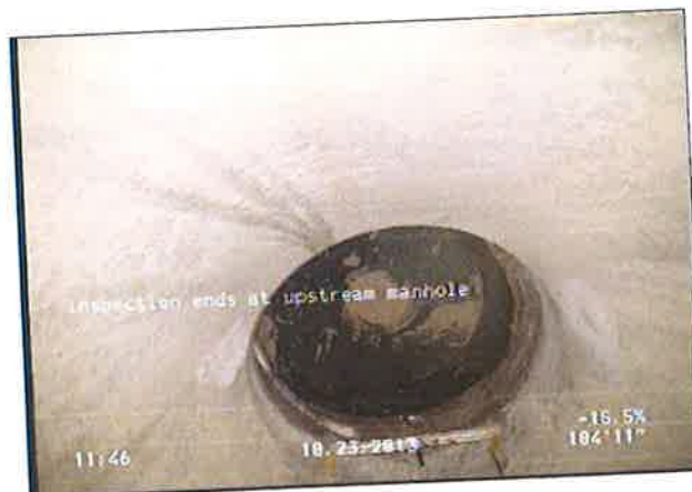
Photo: 10-6_10-5-7_7_23102013_115151_A.JPG inspection ends at upstream manhole
