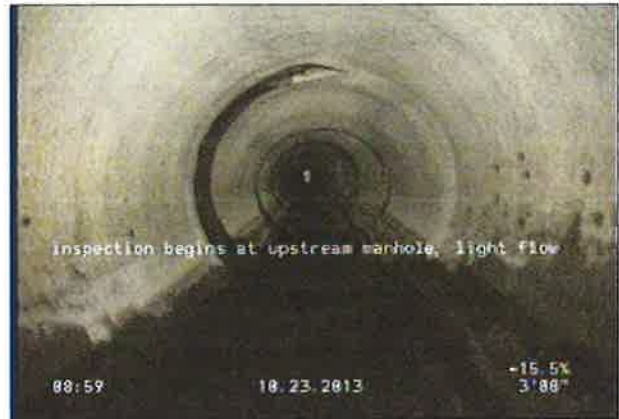
Photo: 10-3_10-4_1_23102013_090500_B.JPG inspection begins at upstream manhole / light flow
