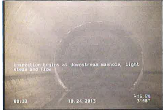
Photo: 10-8-21_10-9_1_24102013_083845_B.JPG inspection begins at downstream manhole / light steam and flow
