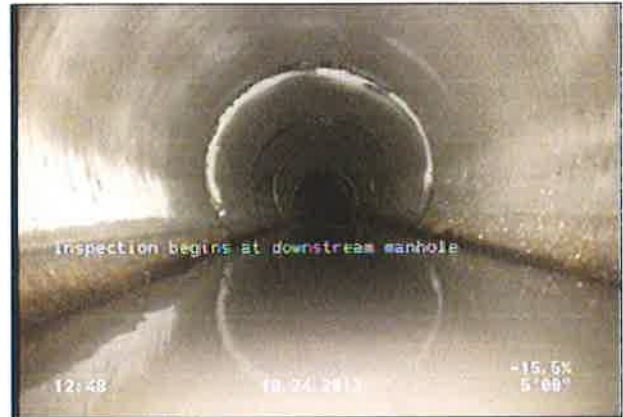
Photo: 10-11-18_10-10-6_1_24102013_125311_B.JPG inspection begins at downstream manhole
