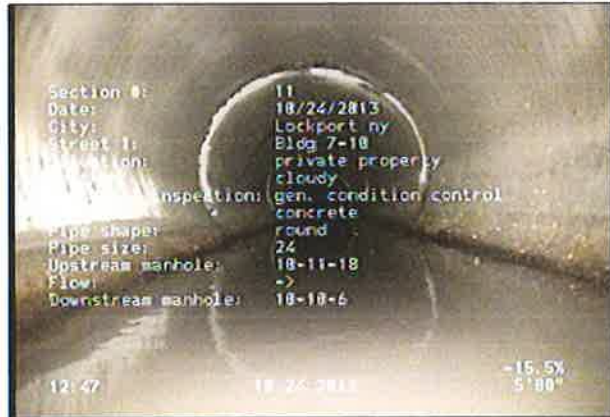
Photo: 10-11-18_10-10-6_1_24102013_125256_A.JPG inspection begins at downstream manhole
