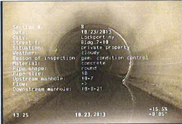
Photo: 10-7_10-8-21_1_23102013_132909_A.JPG inspection begins at upstream manhole
