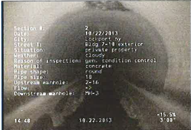
Photo: 2-16_MH-3_1_22102013_145323_A.JPG inspection begins at upstream manhole / Light Flow
