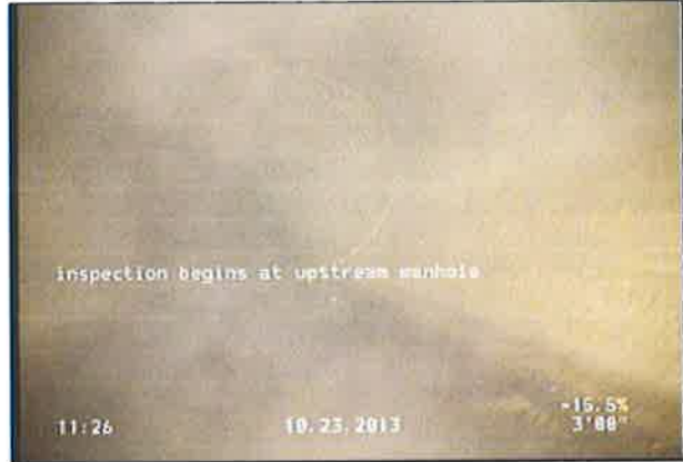
Photo: 10-6_10-5-7_1_23102013_113116_B.JPG inspection begins at upstream manhole
