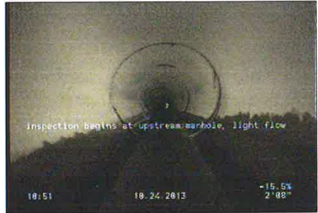
Photo: 10-9_10-10-6_1_24102013_105613_B.JPG inspection begins at upstream manhole / light flow
