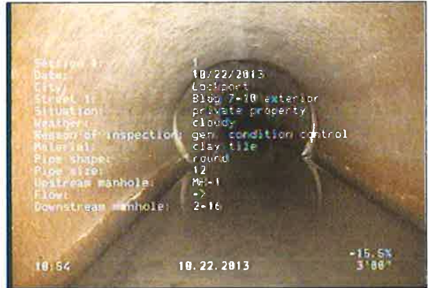
Photo: MH-1_2-16_1_22102013_105953_B.JPG inspection begins at upstream manhole
