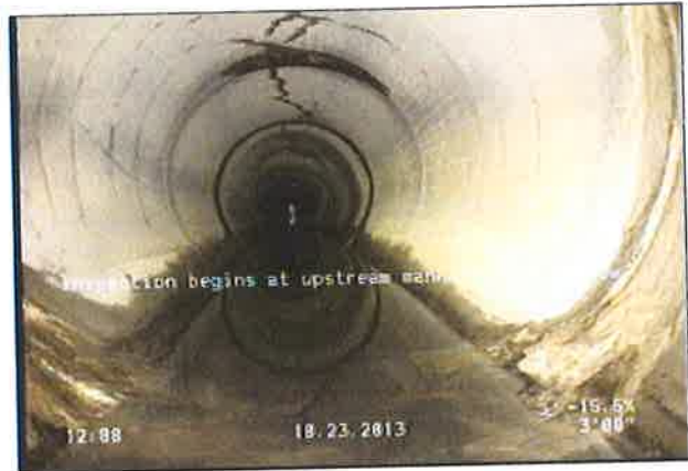
Photo: 10-5-7_10-7-21_1_23102013_121357_B.JPG inspection begins at upstream manhole / light flow
