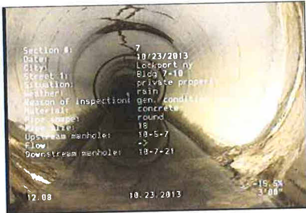
Photo: 10-5-7_10-7-21_1_23102013_121329_A.JPG inspection begins at upstream manhole / light flow
