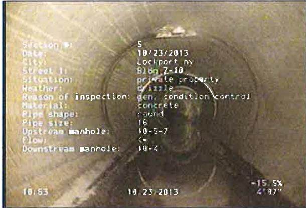
Photo: 10-5-7_10-4_1_23102013_105829_A.JPG inspection begins at downstream manhole / light flow
