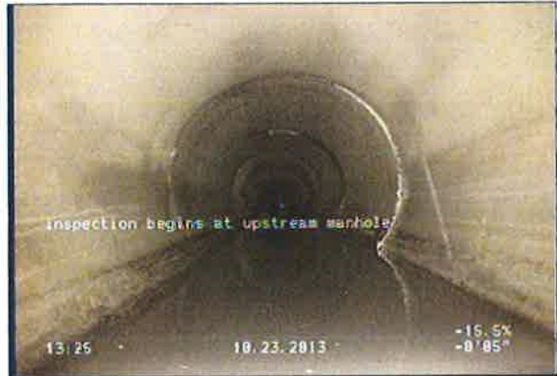
Photo: 10-7_10-8-21_1_23102013_132930_B.JPG inspection begins at upstream manhole
