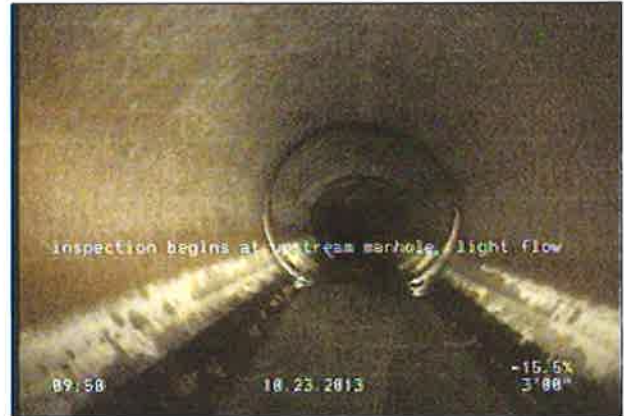
Photo: 10-1_10-2-16_1_23102013_095534_B.JPG inspection begins at upstream manhole / light flow
