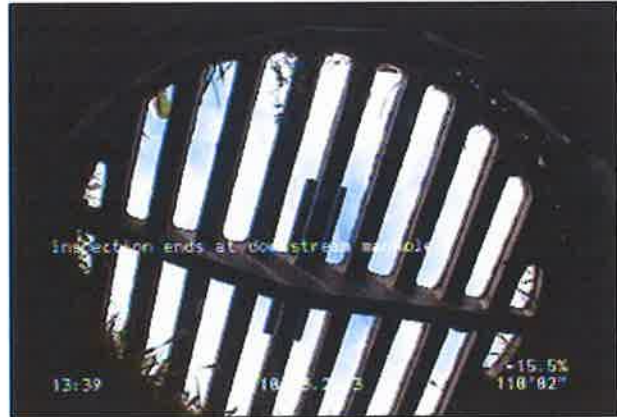
Photo: 10-7_10-8-21_7_23102013_134409_A.JPG inspection ends at downstream manhole
