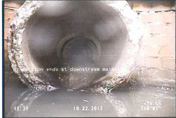
Photo: 2-16_MH-3_44_22102013_154412_A.JPG inspection ends at downstream manhole
