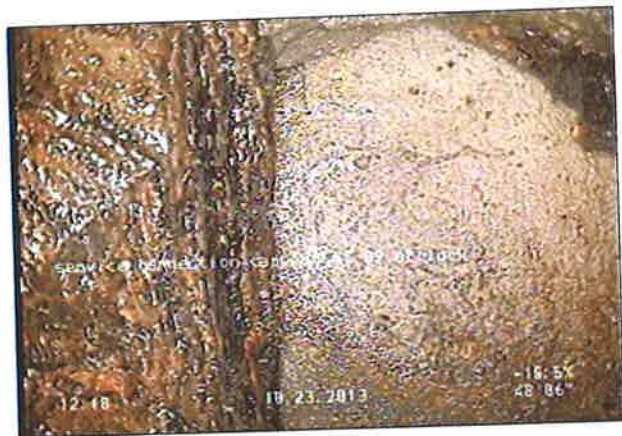
Photo: 10-5-7_10-7-21_7_23102013_122352_A.JPG service connection capped, at 09 o'clock
