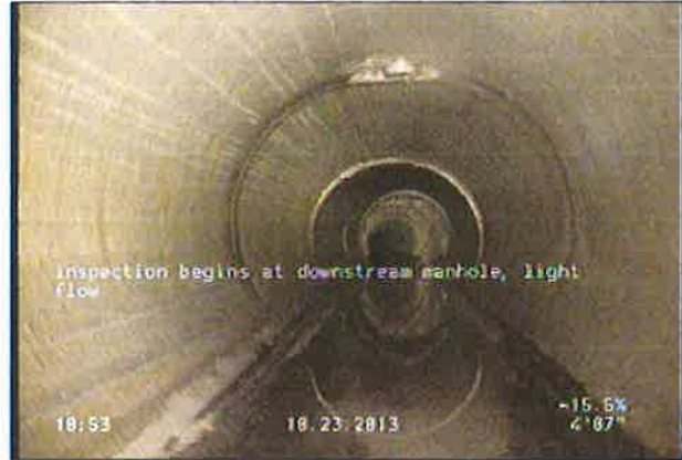
Photo: 10-5-7_10-4_1_23102013_105903_B.JPG inspection begins at downstream manhole / light flow
