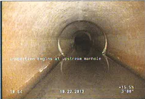
Photo: MH-1_2-16_1_22102013_105946_A.JPG inspection begins at upstream manhole
