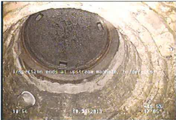
Photo: 10-5-7_10-4_2_23102013_110128_A.JPG inspection ends at upstream manhole / no defects
