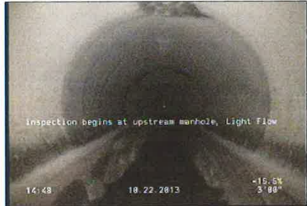
Photo: 2-16_MH-3_1_22102013_145342_B.JPG inspection begins at upstream manhole / Light Flow
