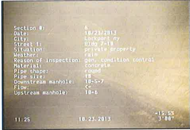
Photo: 10-6_10-5-7_1_23102013_113045_A.JPG inspection begins at upstream manhole
