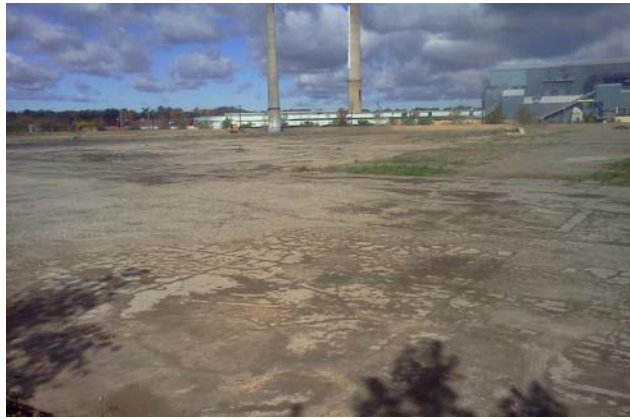
After remediation: south east corner of site
