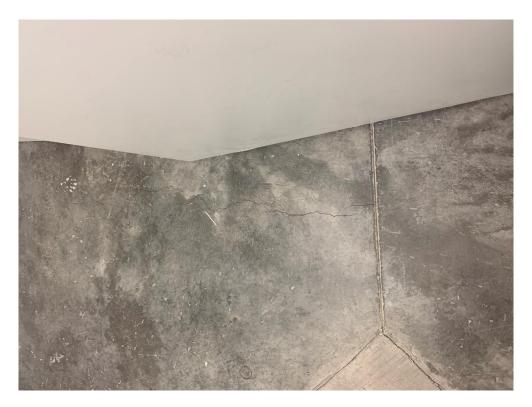
Photograph No. 6 – Minor crack in concrete floor in jail side hallway of the inmate visiting area of the jail.
