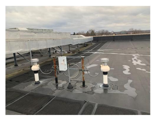
Photograph No. 8 – Sub-slab Depressurization System discharge vents and blowers and power control for discharge vents.
