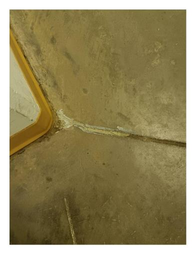
Photograph No. 13 – 2022 Repaired (caulked) crack in concrete floor in men's jail.
