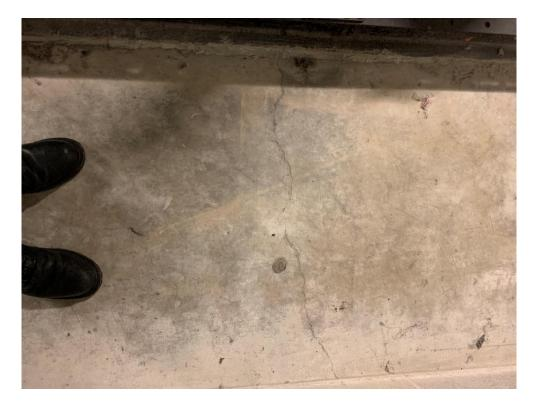
Photograph No. 7 – Minor crack in concrete floor in Room B-37 (i.e. elevator shaft room).
