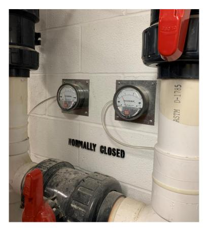
Photograph No. 2 – Sub-slab Depressurization System in basement, depicting pressure gauges.
