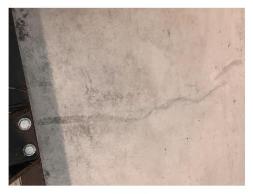
Photograph No. 11 – 2023 Repaired (caulked) crack in concrete floor in Room B-37 (i.e. elevator shaft room).
