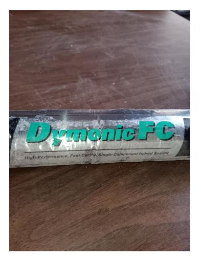
Photograph No. 14 – Caulking used for crack repairs.
