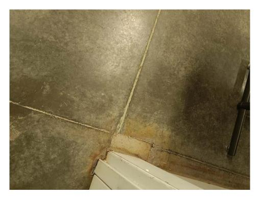
Photograph No. 12 – 2023 Repaired (caulked) crack in concrete floor in jail side hallway of the inmate visiting area of the jail.
