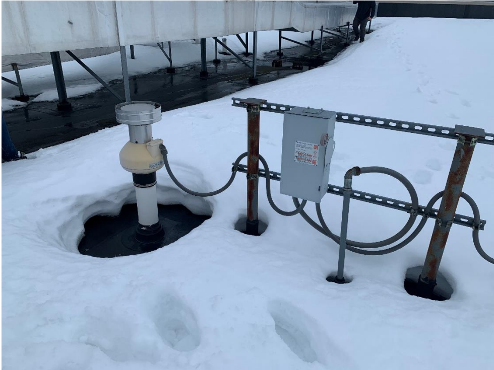
Photograph No. 9 – Roof penetration of southern discharge vent.
