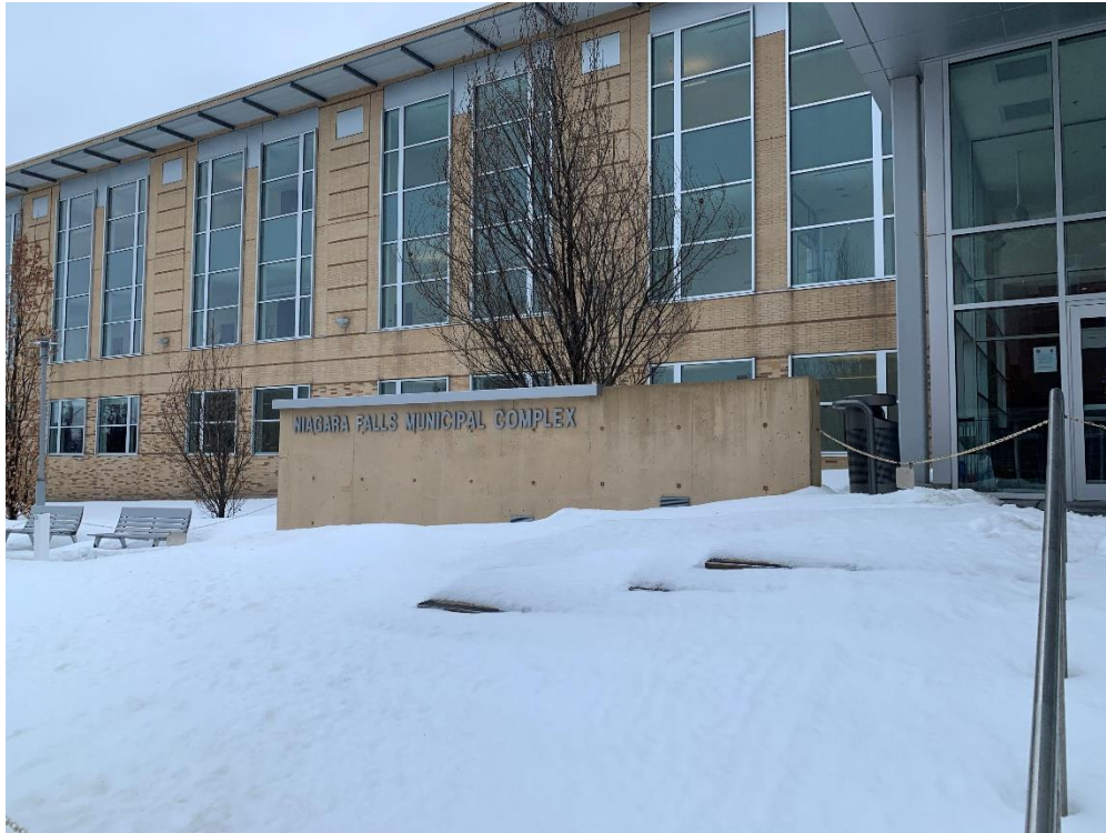
Photograph No. 1 – Front of the Courthouse Building.
