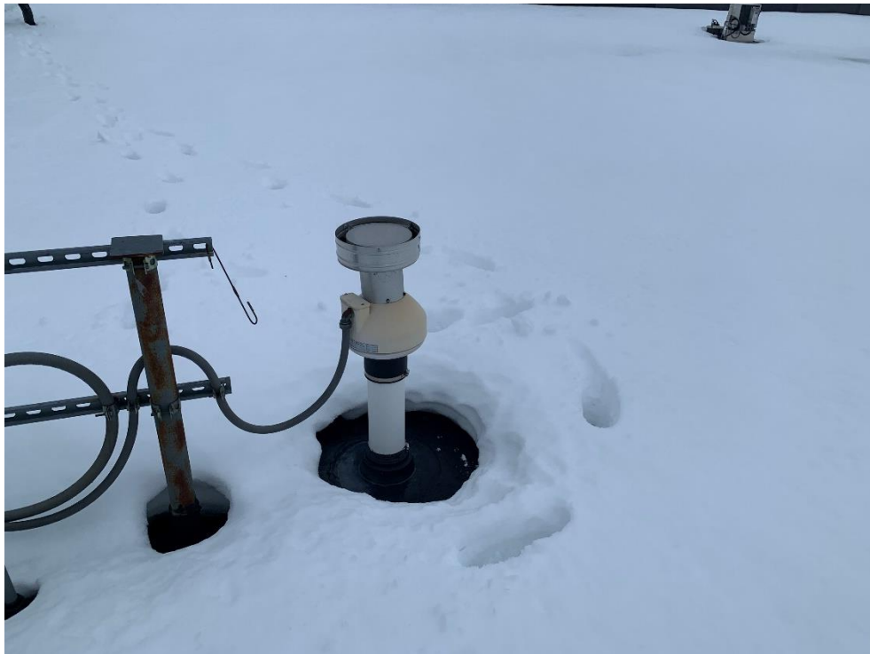
Photograph No. 8 – Roof penetration of northern discharge vent.
