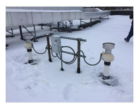
Photograph No. 9 – Sub-slab Depressurization System discharge vents and blowers and power control for discharge vents.
