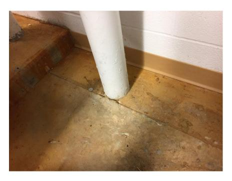
Photograph No. 5 – Sub-slab Depressurization System in basement, depicting stack discharge piping floor penetration.
