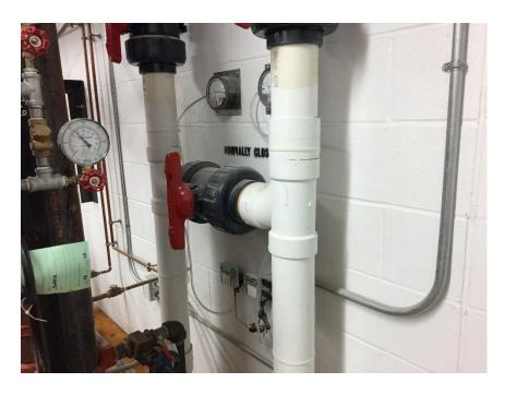
Photograph No. 7 – Sub-slab Depressurization System in basement, depicting alarms and stack discharge piping.
