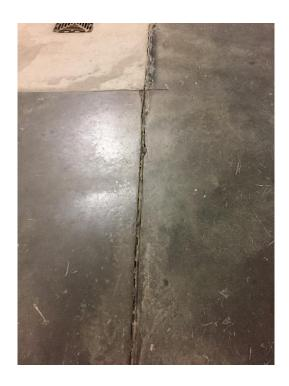
Photograph No. 8 – Floor Joint separation noted at an exposed concrete floor joint within the indoor basement gun range.
