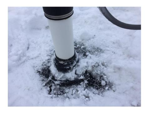
Photograph No. 10 – Roof penetration of southern discharge vent.
