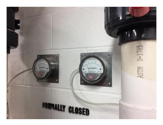
Photograph No. 1 – Sub-slab Depressurization System in basement, depicting pressure gauges.
