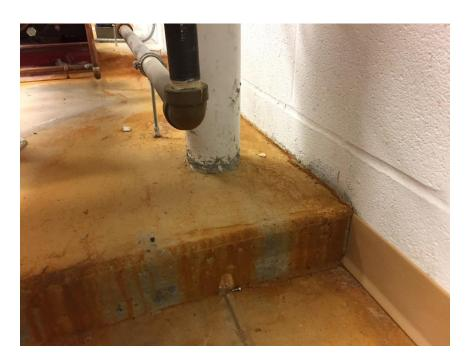
Photograph No. 6 – Sub-slab Depressurization System in basement, depicting stack discharge piping floor penetration.
