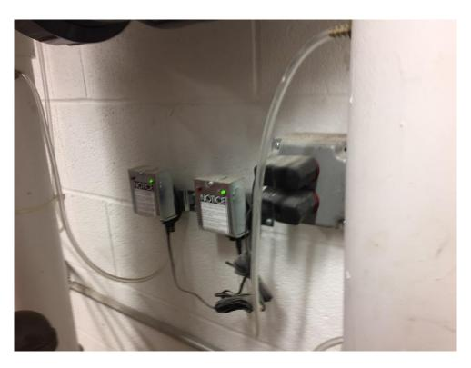
Photograph No. 2 – Sub-slab Depressurization System in basement, depicting alarms.
