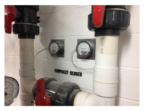
Photograph No. 4 – Sub-slab Depressurization System in basement, depicting pressure gauges.
