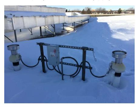
Photograph No. 6 – Sub-slab Depressurization System discharge vents and blowers and power control for discharge vents.
