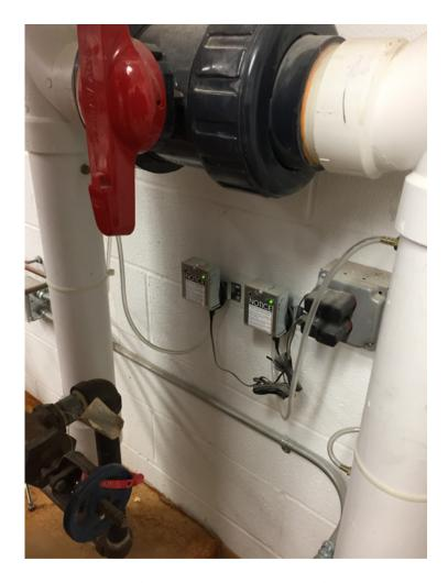
Photograph No. 5 – Sub-slab Depressurization System in basement, depicting alarms and stack discharge piping.
