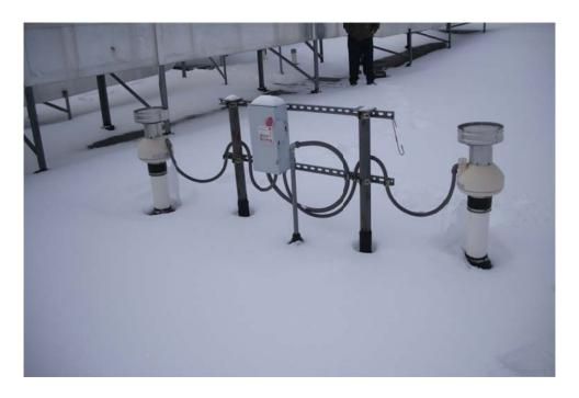
Photograph No. 5 – Sub-slab Depressurization System discharge vents and blowers.
