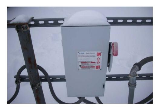
Photograph No. 6 – Sub-slab Depressurization System power control for discharge vents.
