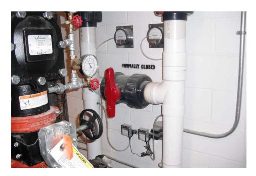
Photograph No. 4 – Sub-slab Depressurization System in basement, depicting alarms, pressure gauges and stack discharge piping.
