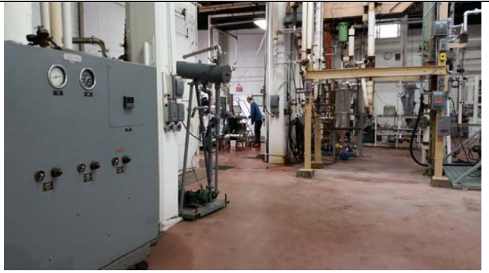
Site Building 3 testing area
