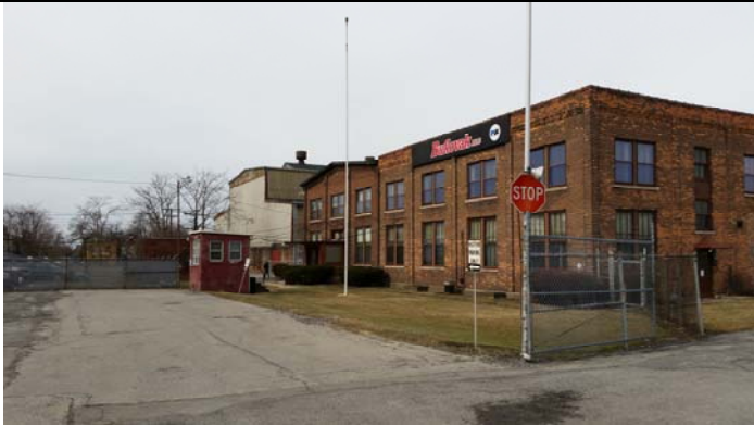
South side of Site Building 1
