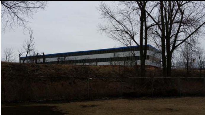
North adjacent property
