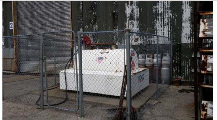
AST south of Storage Building & Receiving portion of Site Building 2
