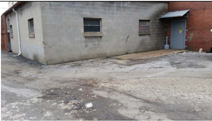
Area at north end of 10,000-gallon UST closed in place
