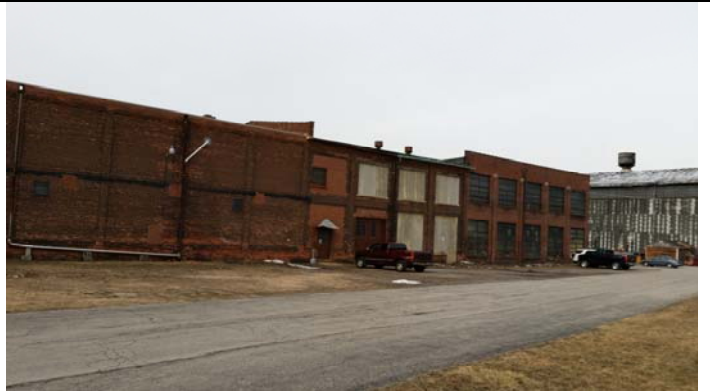
East side of Site Building 1
