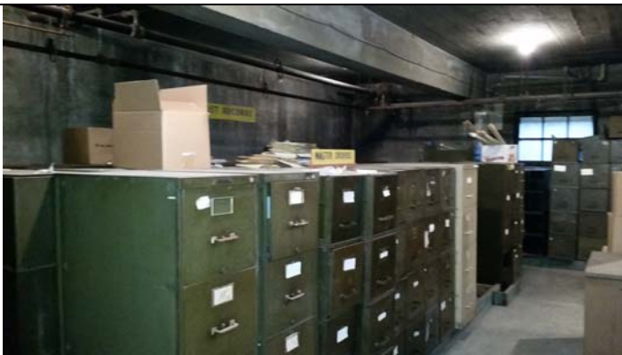
Basement of Site Building 1
