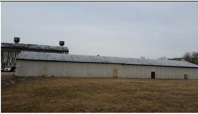
South side of Site Building 4
