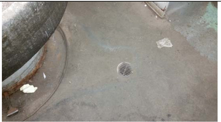
Floor drain in restroom in Site Building 2
