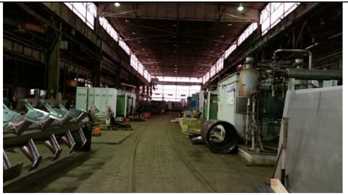
Main Floor Fabrication portion of Site Building 2
