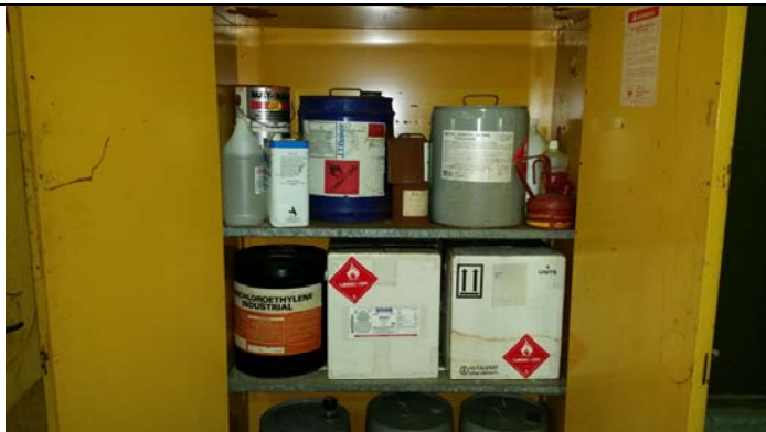
Flammable Cabinet chemical storage in Site Building 3
