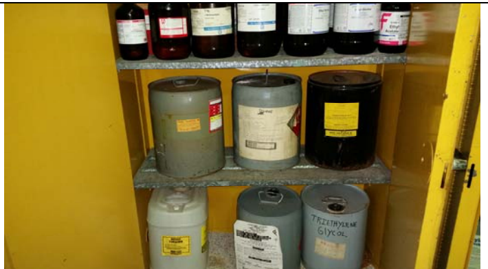
Flammable Cabinet chemical storage in Site Building 3
