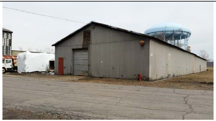
West side of Site Building 4
