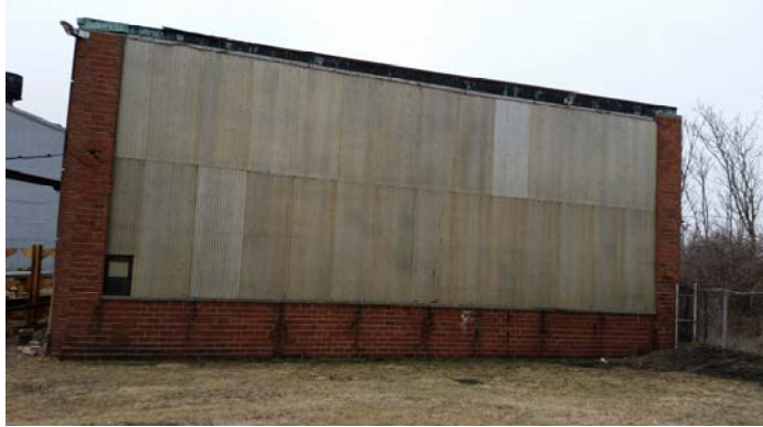
East side of Site Building 2
