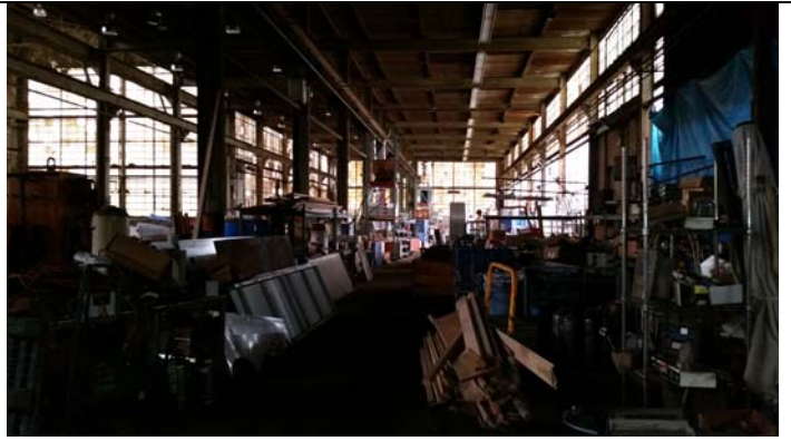
Fabricating Department portion of Site Building 2 used as storage
