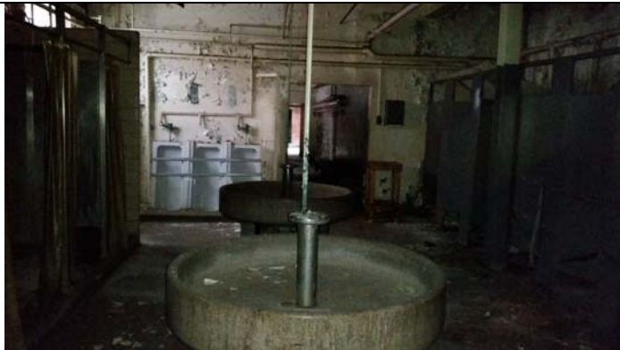
Locker room area in Site Building 2
