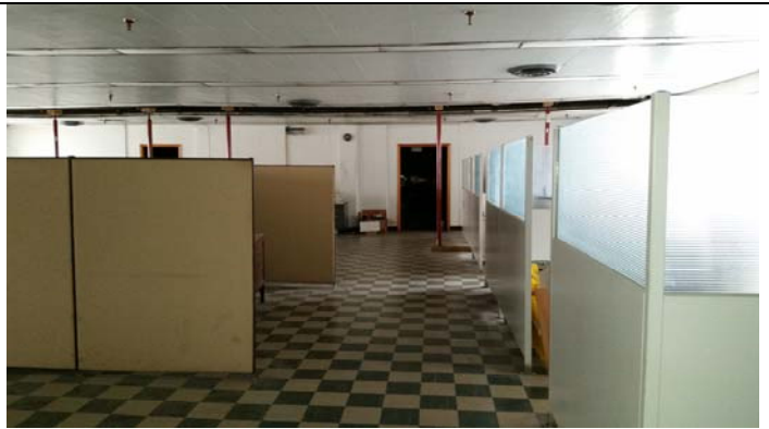
Second floor of Site Building 1
