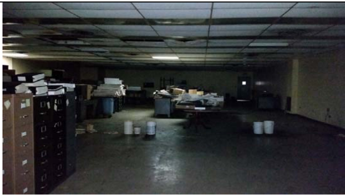
Second floor of Site Building 1
