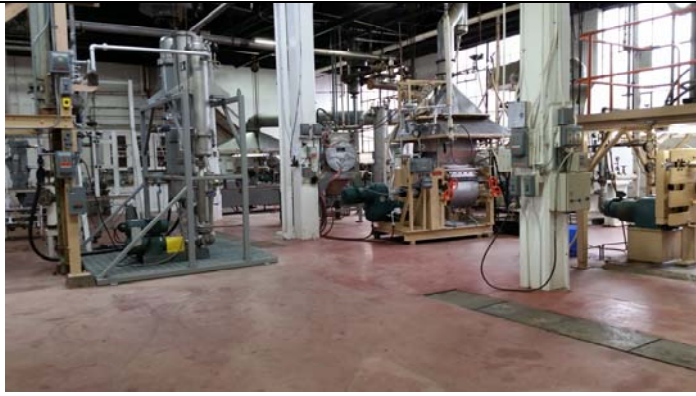
Site Building 3 testing area
