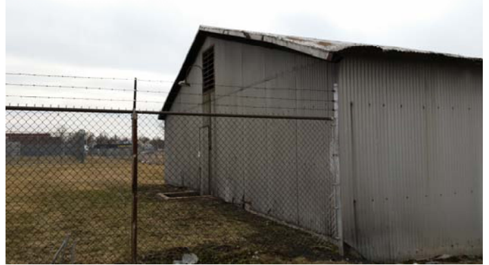
East side of Site Building 4
