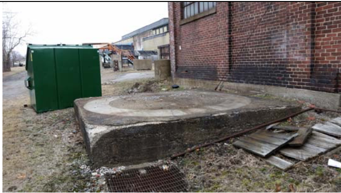
Pad for former chimney
