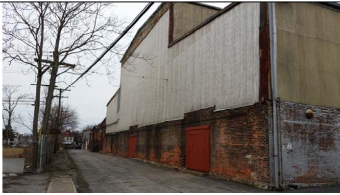
South side of Site Building 2
