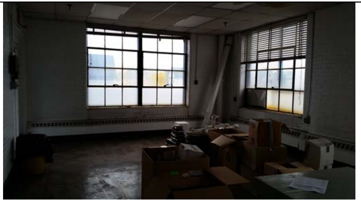
Office space on second floor of Site Building 3
