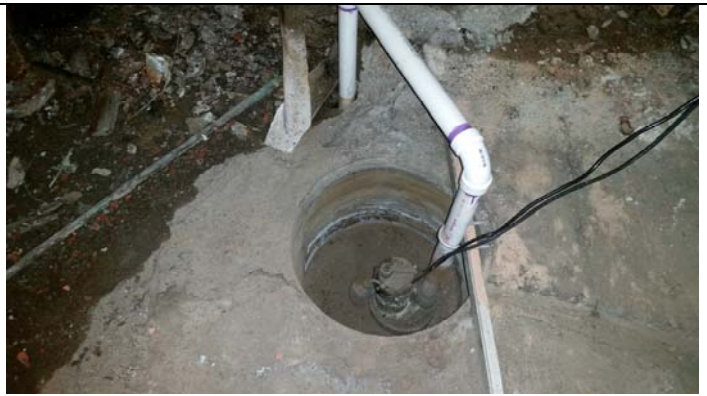
Sump in basement of Site Building 1
