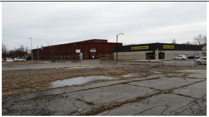
South adjacent properties
