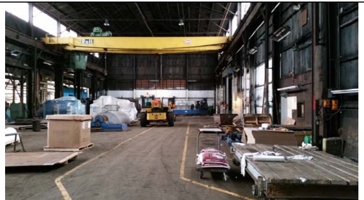
Storage Building & Receiving portion of Site Building 2
