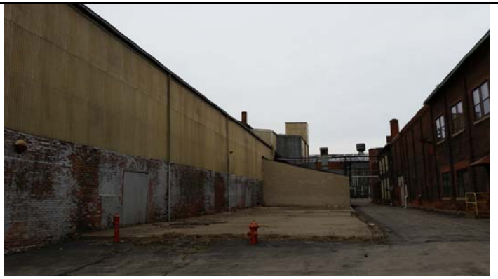
East side of Site Building 2
