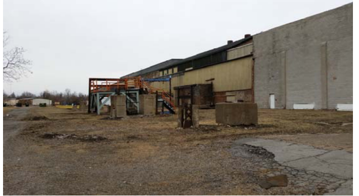
West side of Site Building 2
