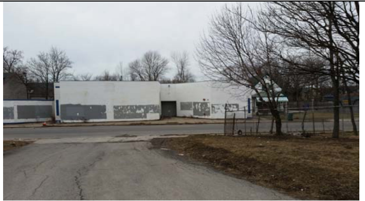
West adjacent property
