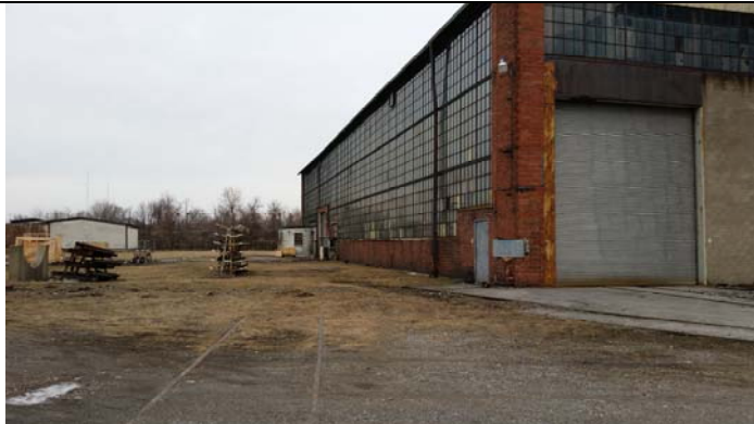
West side of Site Building 2
