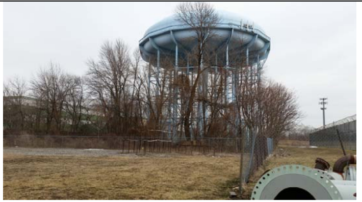
East adjoining property
