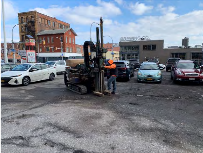
Boring B11 Location
