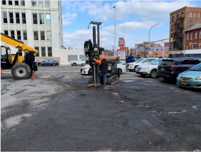
Boring B13 Location
