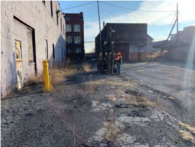
Boring B16 Location
