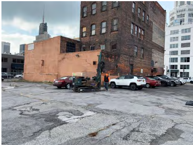
Boring B10 Location
