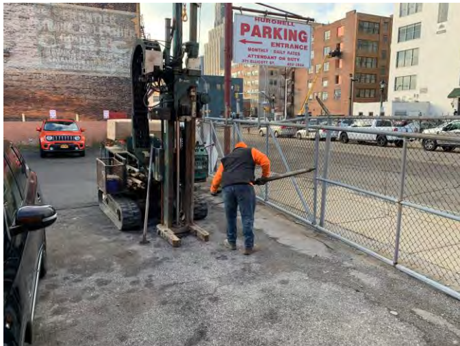
Boring B4 Location
