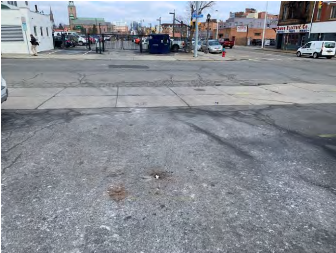
Boring B12 Location
