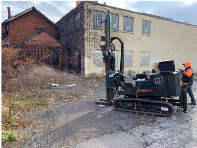
Boring B7 Location
