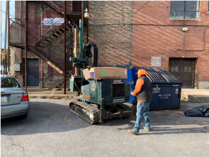
Boring B14 Location
