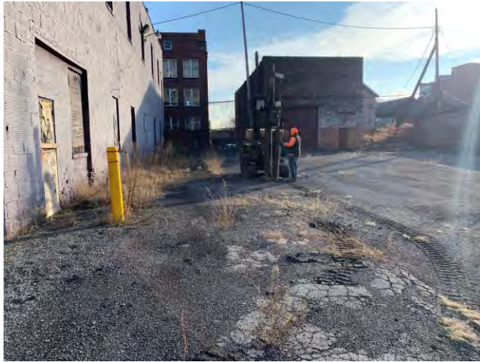
Boring B3 Location
