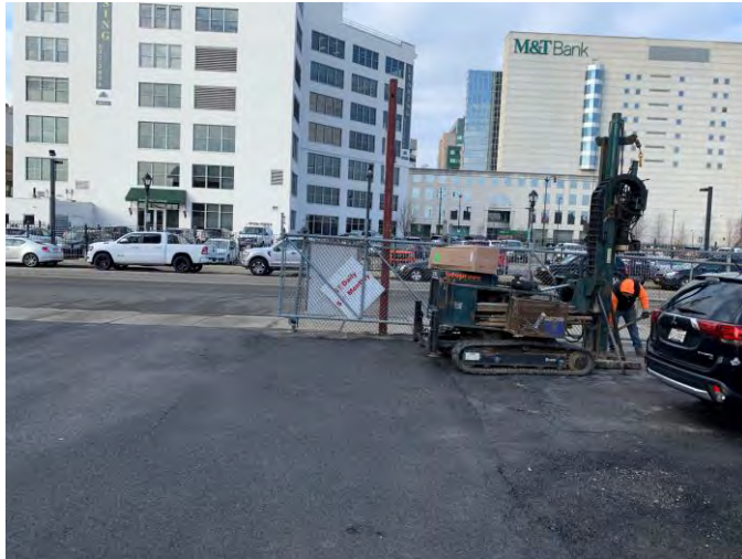
Boring B5 Location
