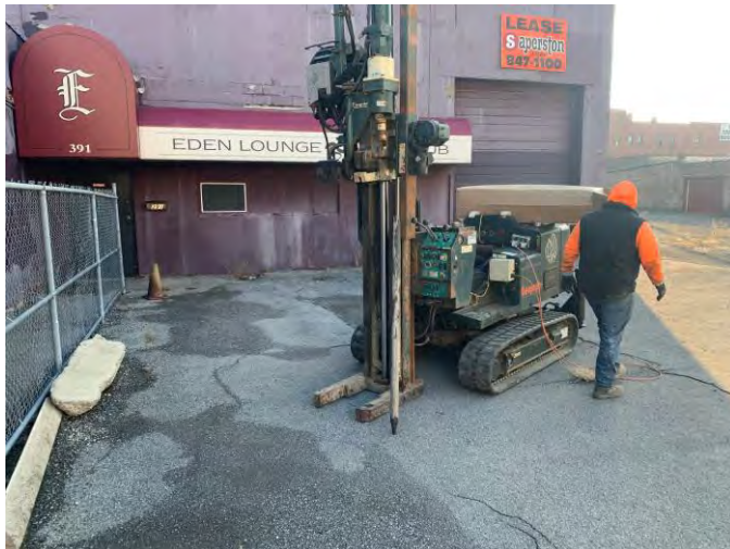
Boring B2 Location
