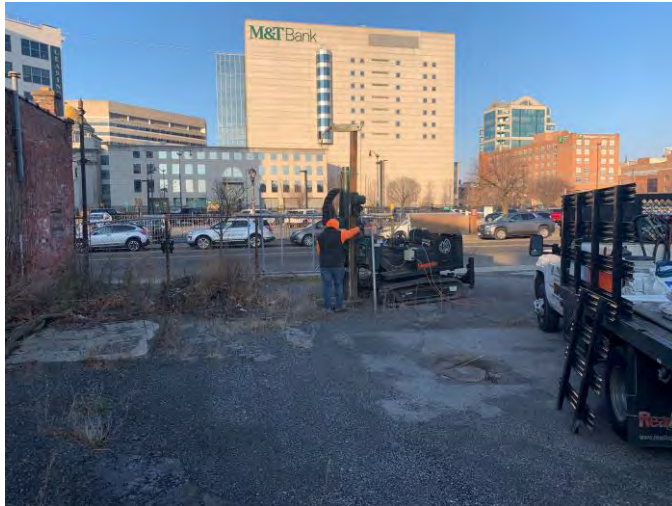
Boring B1 Location
