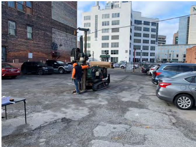
Boring B6 Location
